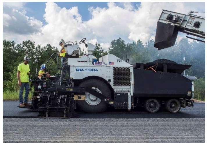
SMA thin overlay being placed over an intermediate layer.
