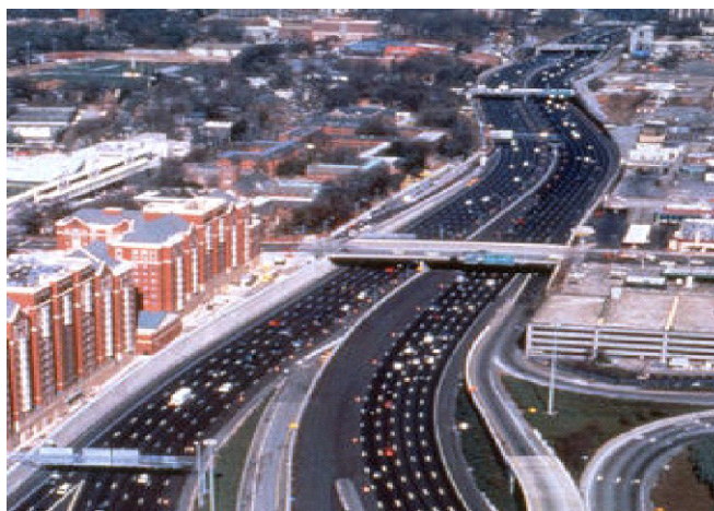
Figure 2: SMA HOV lane construction project in Atlanta. (Source: GDOT)
