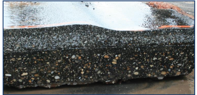
Figure 10: Partial slab from a rutted SMA project. (Source: Alabama DOT)
