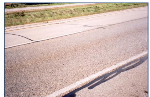
Figure 3: A concrete pavement overlay in Wisconsin after eight years. (Source: National Center for Asphalt Technology (NCAT))
