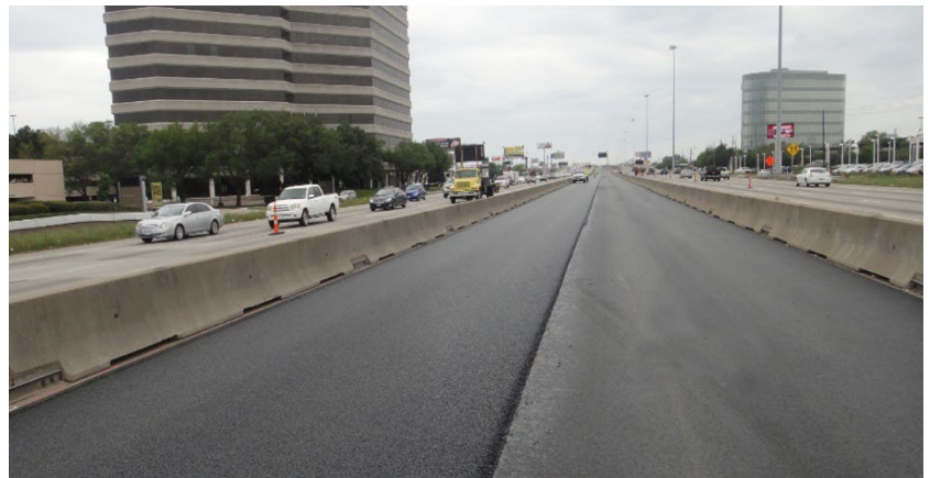
Crack attenuating mix on Houston's IH-69 project. Source: Tom Scullion, Texas A&M Transportation Institute
