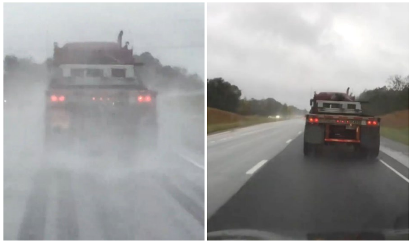
Reduced splash and spray and improved visibility on OGFC section. Source: National Center for Asphalt Technology
