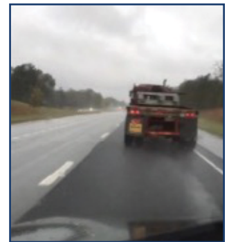
Figure 2. Reduction of backsplash on an OGFC. (Source: Watson et al. 2018)
