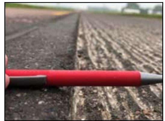
Figure 12. Micromilled surface. (Source: MnDOT)
