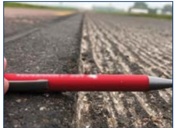
Figure 5. ¼-inch UTBWC on a micro-milled surface. (Source: MnDOT)
