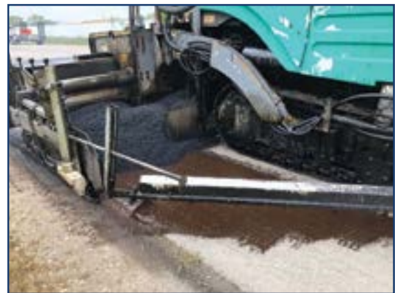
Figure 1. UTBWC is applied using a spray paver. (Source: MnDOT)
