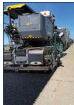
Figure 3. Freshly placed uncompacted UTBWC. (Source: Asphalt Surface Technologies Corp.)
