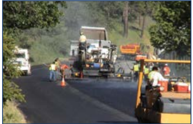
Figure 14. UTBWC rolling operations. (Source: Caltrans)
