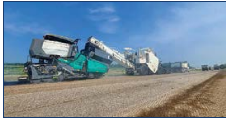
Figure 13. Use of MTV and spray-paver. (Source: Asphalt Surface Technologies Corporation.)
