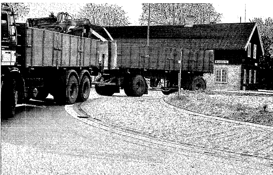
In this little roundabout part of the carriageway (the so-called short-cut-area) is paved with paving stones that the cars will try to avoid but which lorries can pass.
