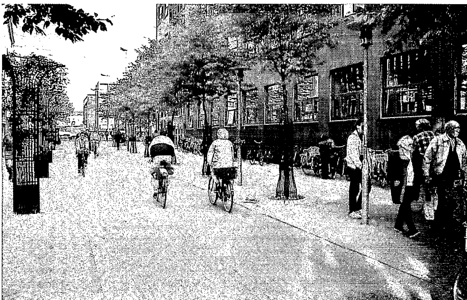
The cyclists' track area is marked with brown hard burned paving bricks in stretcher bond while the rest of the area is paved in yellow hard burned bricks.
