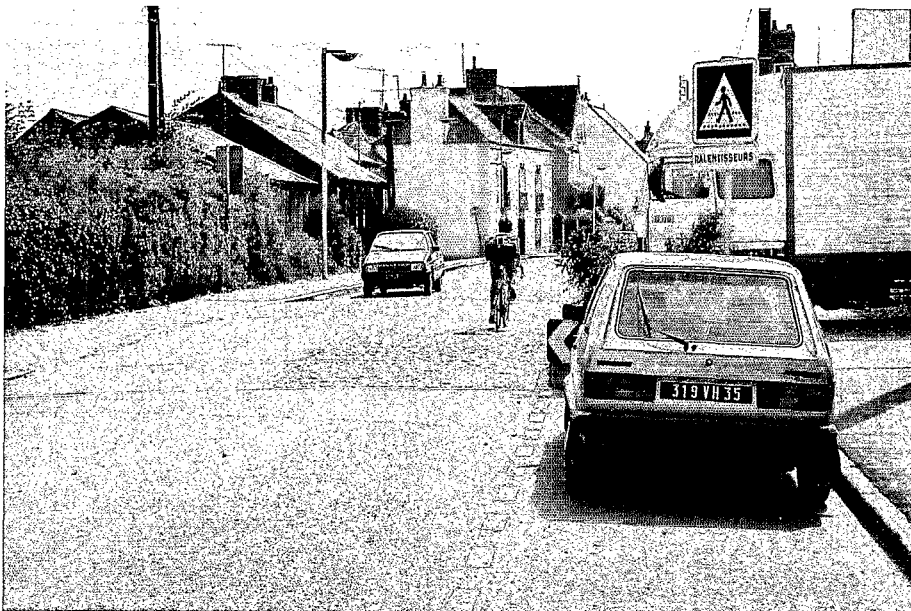
The 6 m wide carriageway of the old highway is diversified by changed road surfaces and a raised area.
