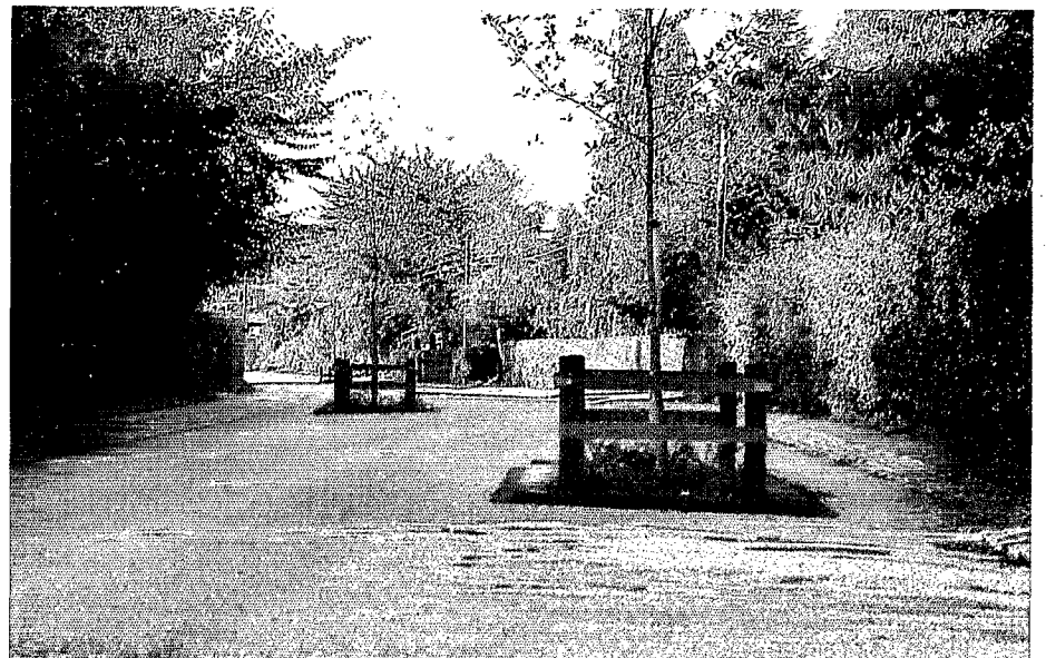
Staggering with narrowing.
