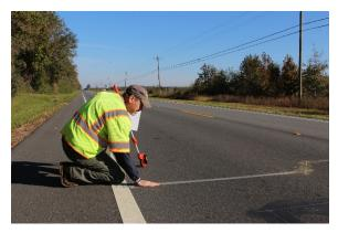
Figure 9 – WIM Sensor Inspection
