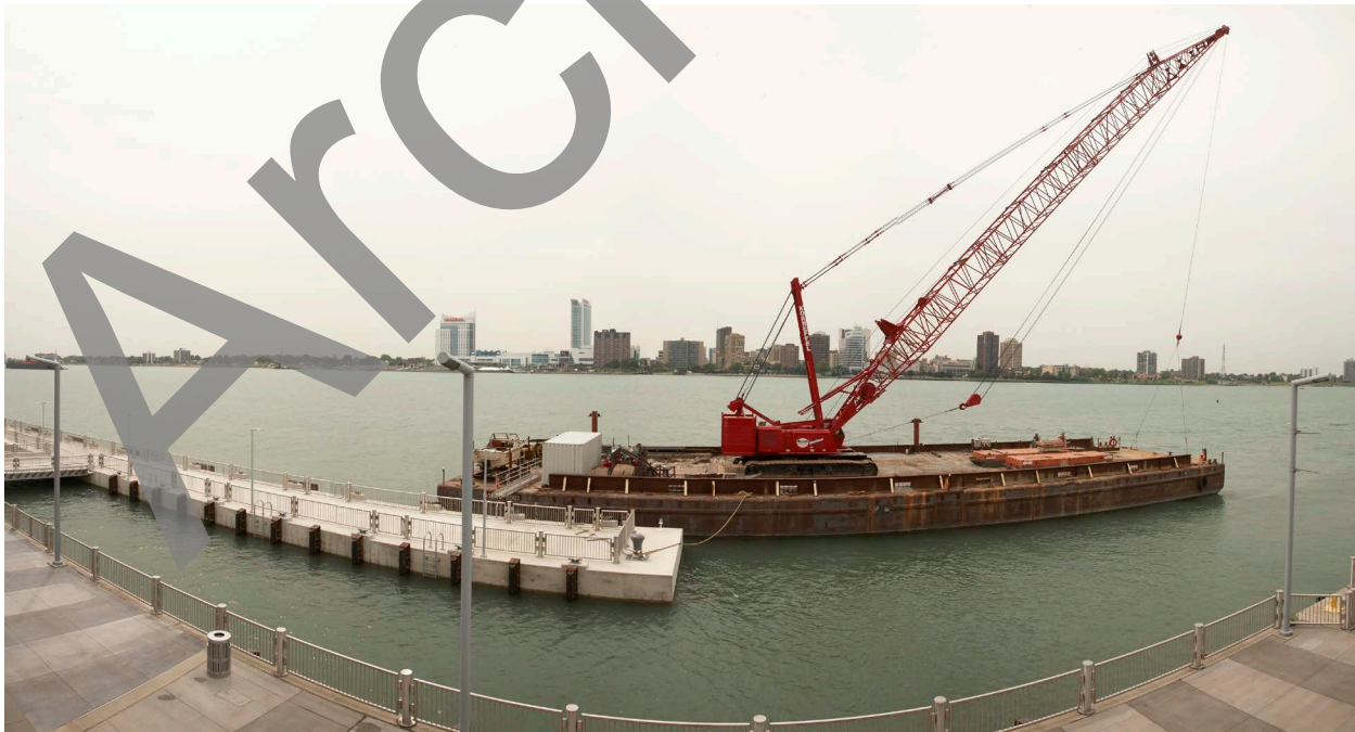
Wharf and Seawall were generally constructed from barges as self-perform by Korneffel.
