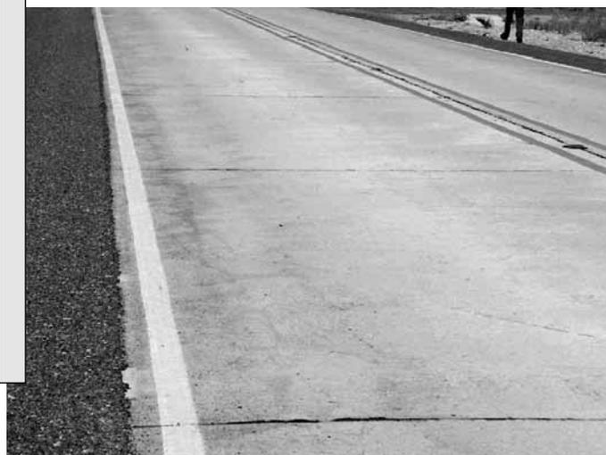
LTPP pavement rehabilitation experiments included jointed concrete pavements.
