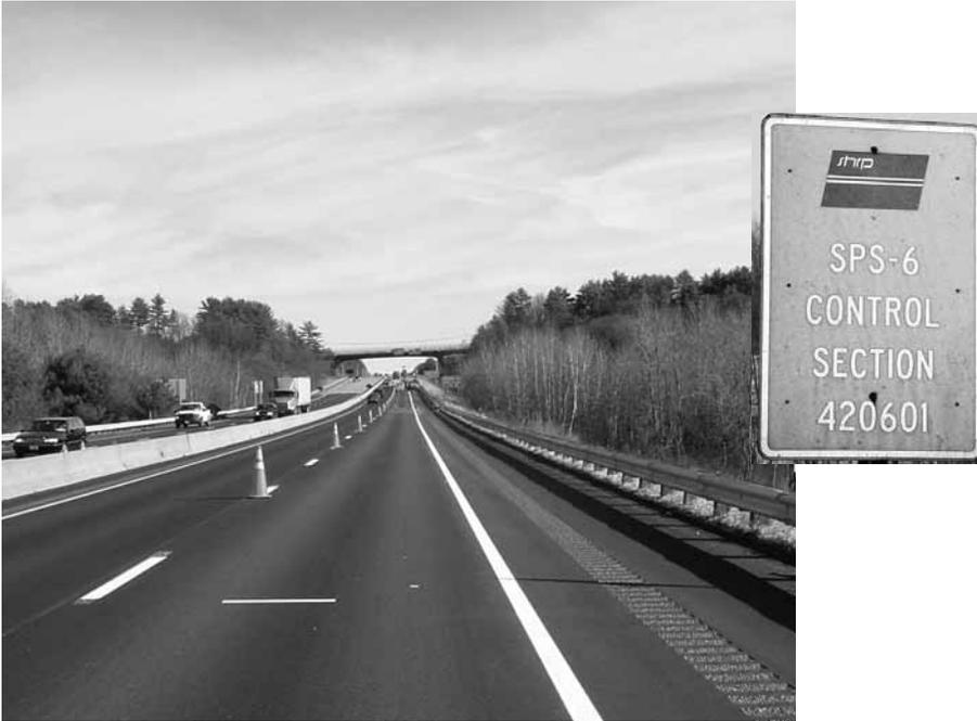
The LTPP program's SPS-5 and SPS-6 experiments examined rehabilitation strategies for both flexible and rigid pavements.
