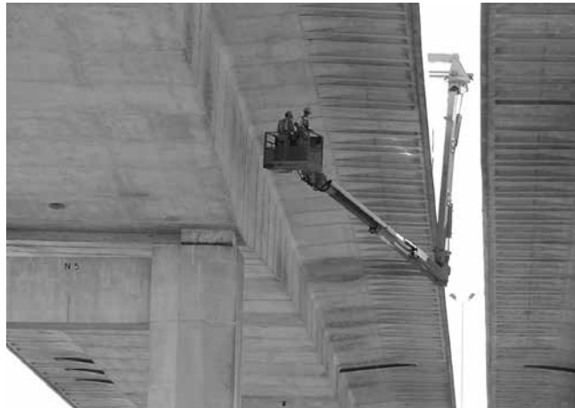
A bridge inspection is conducted by the Michigan Department of Transportation.
