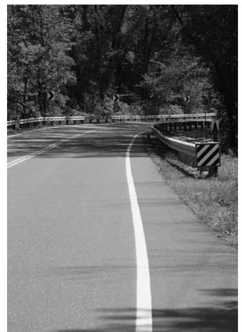
The All-Weather Pavement Marking System makes it easier for drivers to see markings on wet roads.
