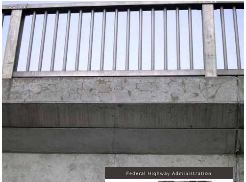
The edge beam supporting this bridge railing has minor ASR-related cracking.
