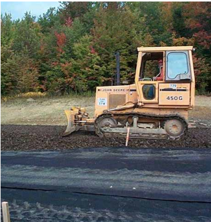
Tire-derived aggregate made from recycled tires is applied to a roadway.
