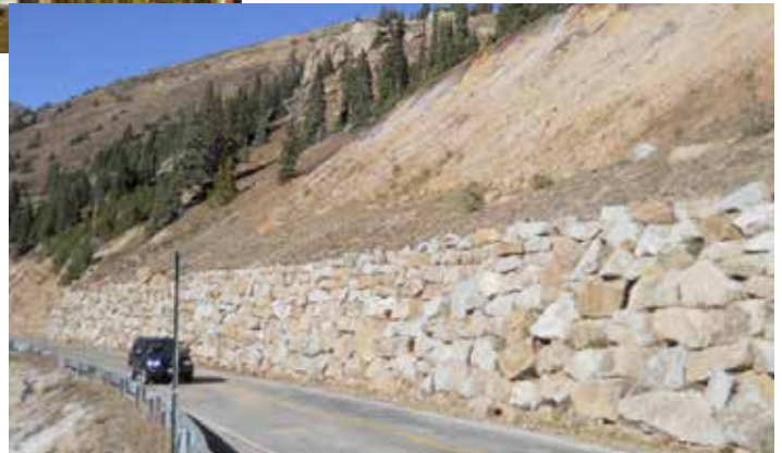
Top: A repair is made to Hanging Lake Tunnel along I-70, near Glenwood Springs, CO. Right: A rockery wall at the toe of a scaled rock and soil cut slope along Guanella Pass Road near Georgetown, CO. Left: Damage to a culvert on I-70 and adjacent embankment that have failed near the Eisenhower Tunnel in CO.
