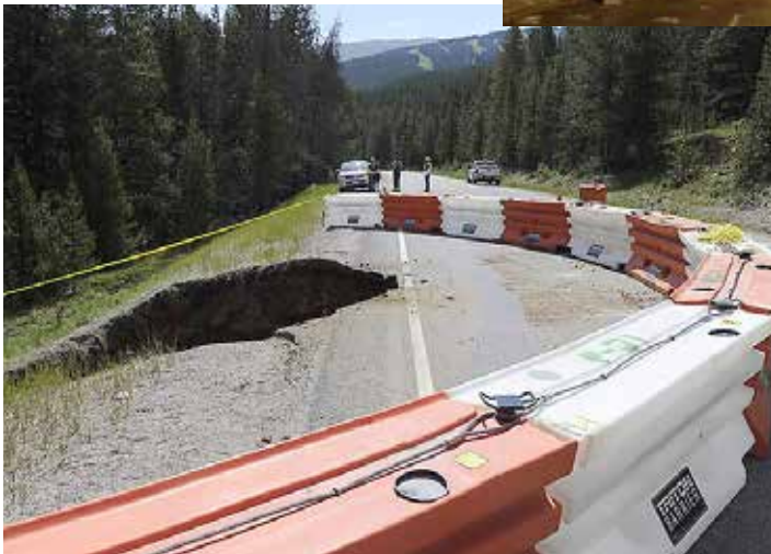
Top: A repair is made to Hanging Lake Tunnel along I-70, near Glenwood Springs, CO. Right: A rockery wall at the toe of a scaled rock and soil cut slope along Guanella Pass Road near Georgetown, CO. Left: Damage to a culvert on I-70 and adjacent embankment that have failed near the Eisenhower Tunnel in CO.
