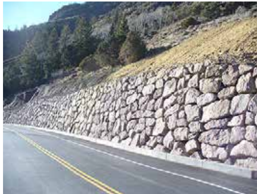
FHWA used rockeries to improve safety and reduce maintenance needs when reconstructing part of the Beaver to Junction Highway in southern Utah.
