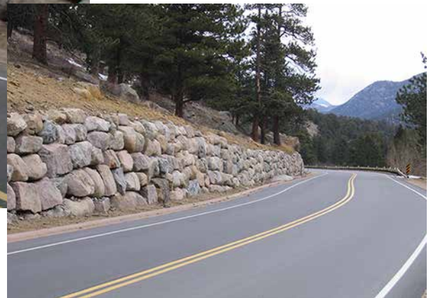
Rockerries built by FHWA on Bear Lake Road in Colorado's Rocky Mountain National Park have improved both safety and aesthetics.
