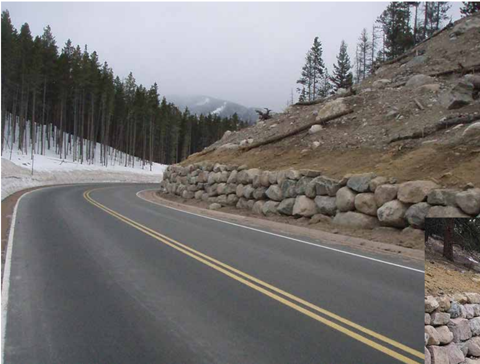
Rockerries built by FHWA on Bear Lake Road in Colorado's Rocky Mountain National Park have improved both safety and aesthetics.
