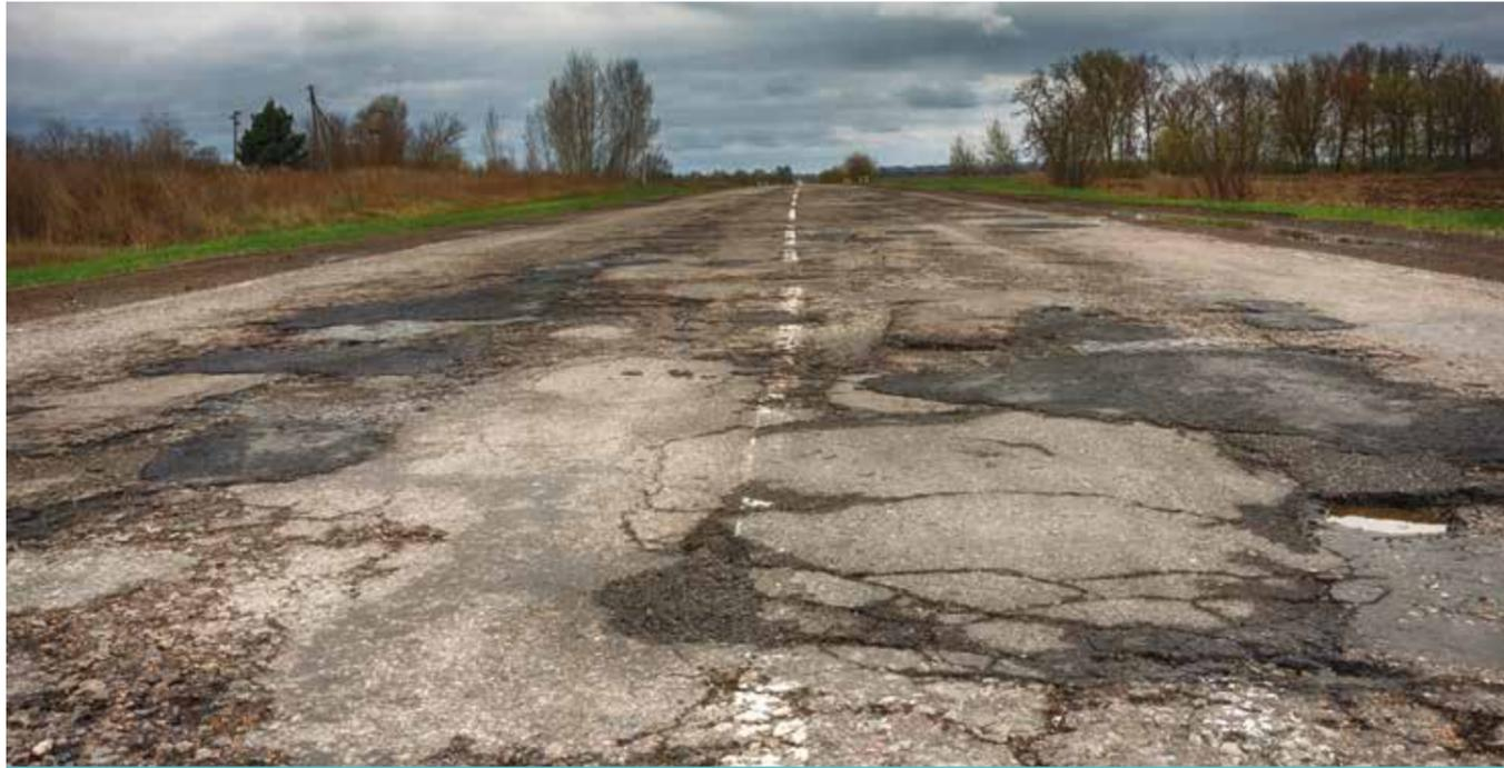
Figure 7. Photo. Example of severe pavement surface cracks and spiraling caused by weather conditions and vehicle weight wear and tear over time. ©undefined/iStock.
