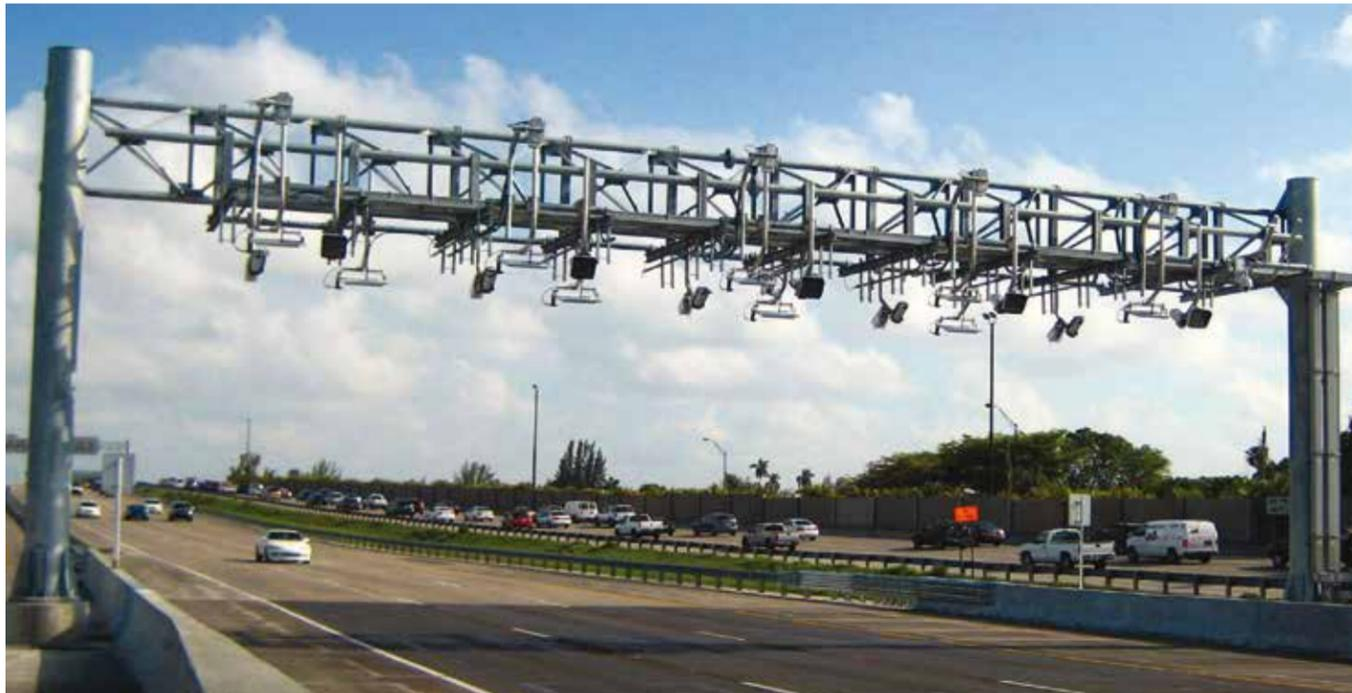
Figure 4. Photo. Transponders and cameras built into overhead gantry automate data gathering and toll collection while vehicles move at highway speed. ©Florida's Turnpike Enterprise.
