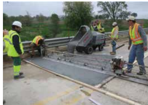
Figure 10. UHPC overlay installation on the westbound lane. (2)
