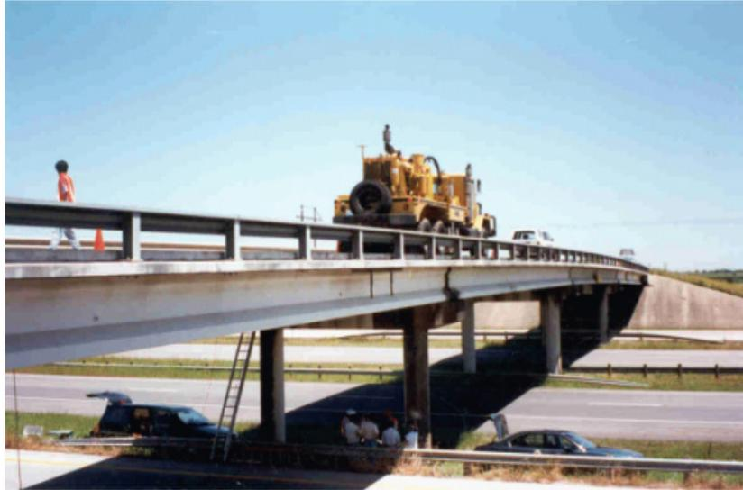
Figure 33. Photo. Vibroseis truck over west pier of Woodville Road Bridge.
