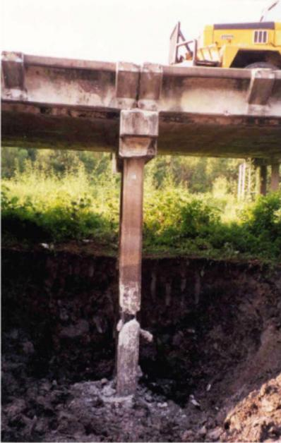
Figure 31. Photo. Sheared south pile of bent 12.
