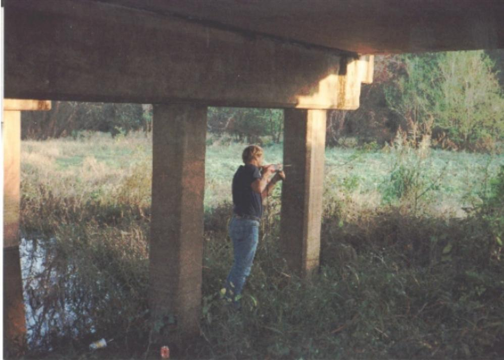
Figure 14. Photo. Drilling concrete holes to mount seismic accelerometers on bent 2 of structure 4, Trinity River Relief Bridge.
