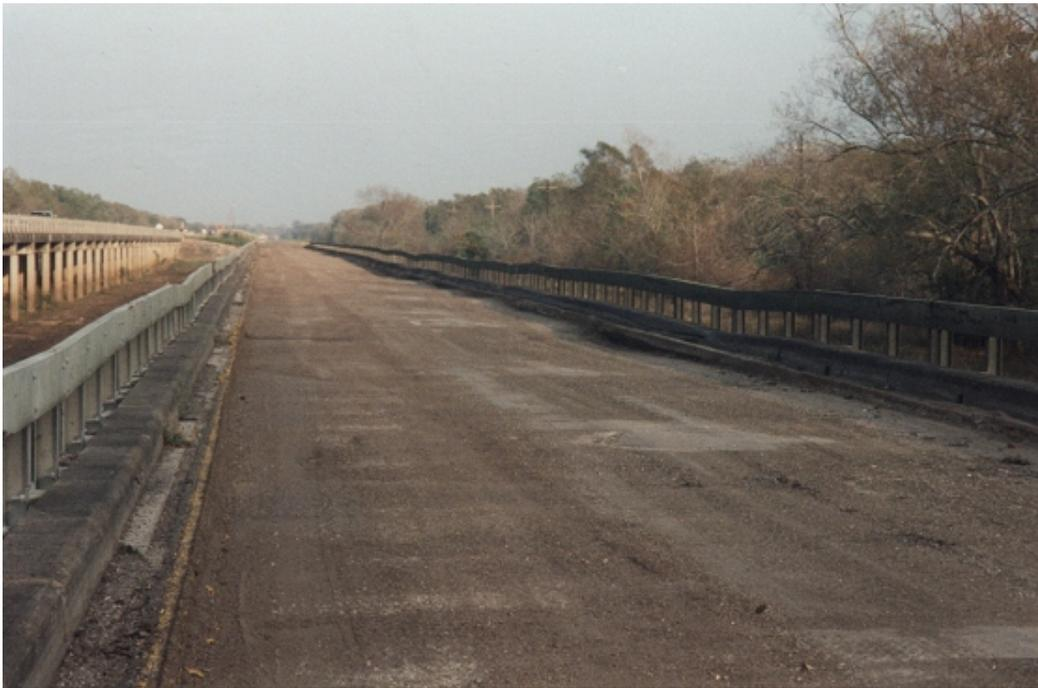
Figure 4. Photo. Excessive differential settlements on relief structure 4, Trinity River Relief Bridge.
