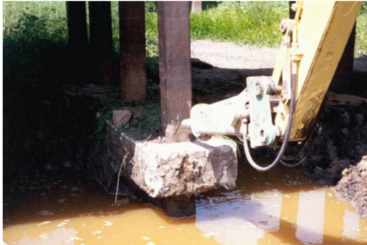
Figure 27. Photo. Shearing of pile of bent 2.
