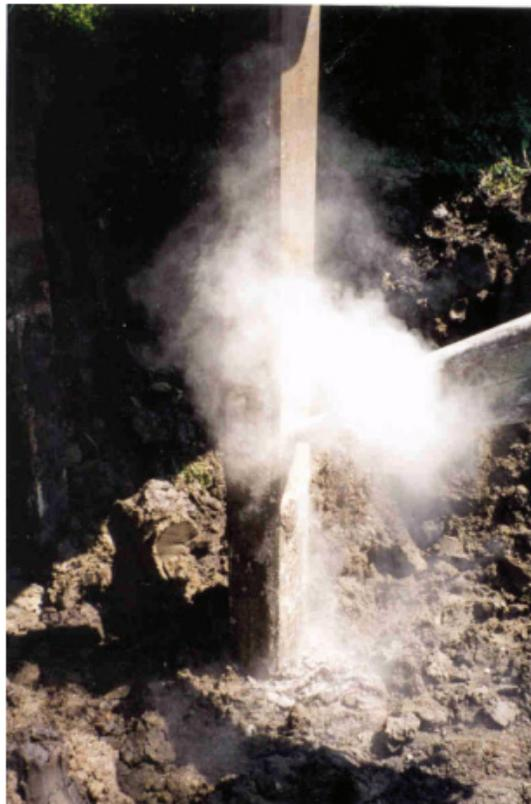
Figure 28. Photo. Shearing of pile of bent 12.
