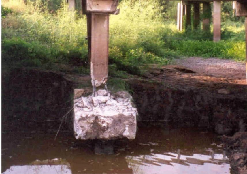
Figure 29. Photo. Sheared south pile of bent 2 with ground water seepage.
