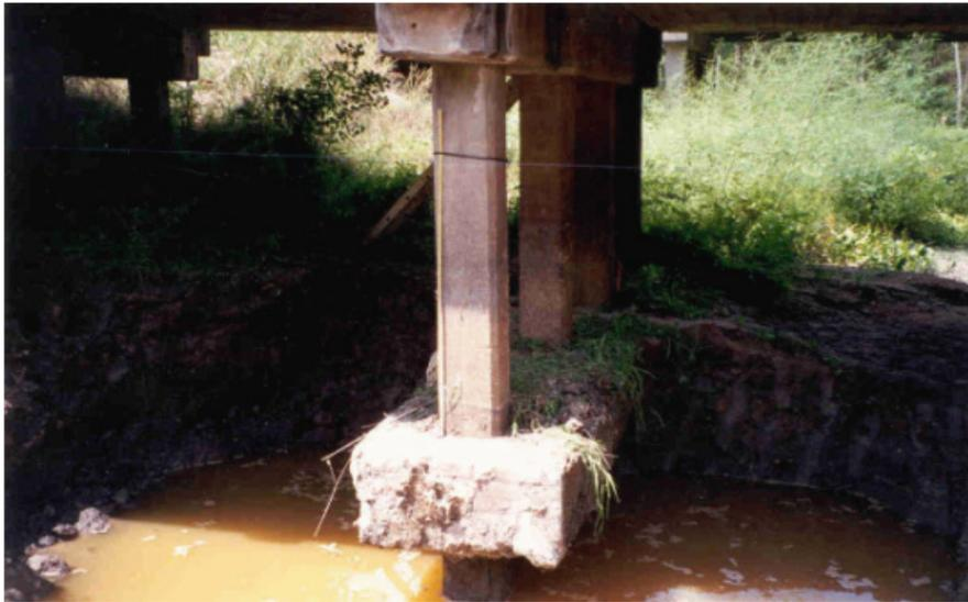
Figure 24. Photo. Ground water in excavation of bent 2, Trinity River Relief Bridge.
