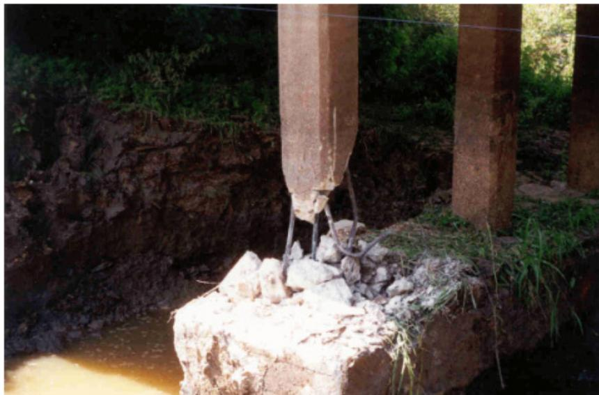
Figure 30. Photo. Bent and broken rebars of south column of bent 2.
