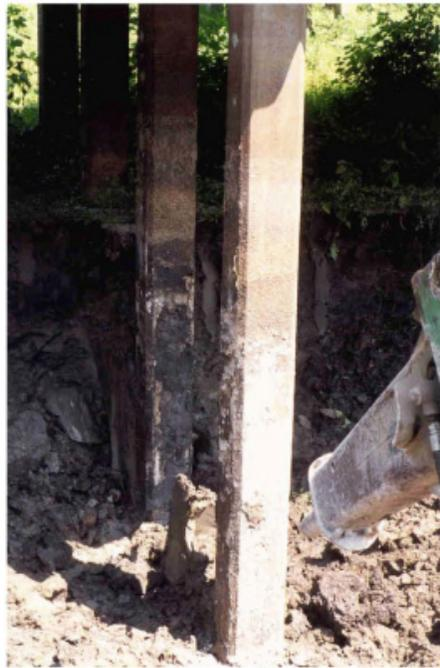
Figure 26. Photo. Piles of bent 12 just after excavation.
