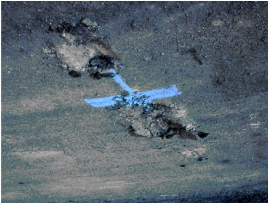
Figure 19. Photo. Dual-wheel depressions in asphalt overlay on deck over bent 2.
