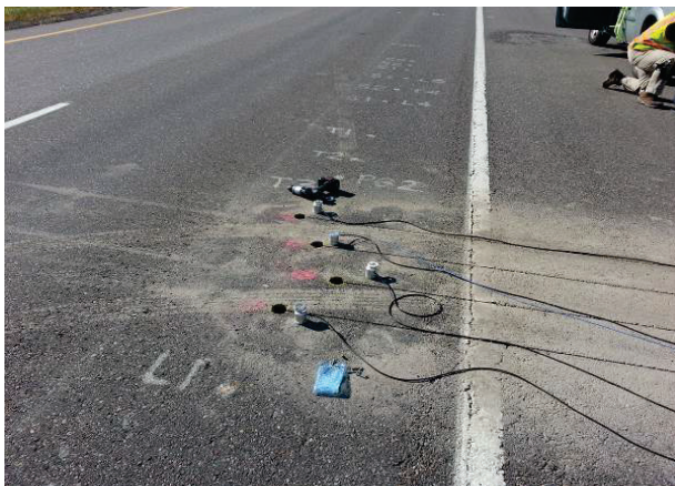
Figure 27. Photo. Grooving of pavement for sensor installation.
