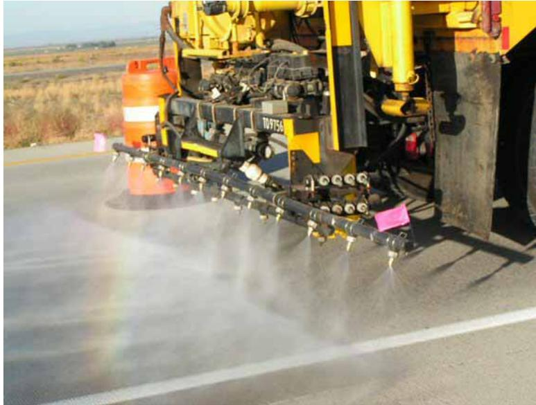
**Figure 20. Spraying 30 percent LiNO<sub>3</sub> solution with a tanker truck on a concrete pavement near Mountain Home, ID.**
