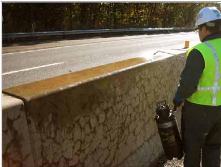
**Figure 21. Spraying 30-percent LiNO<sub>3</sub> solution with handheld spray applicator on barrier wall near Leominster, MA.**
