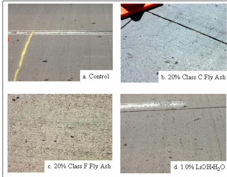
**Figure 18. Photographs of 12-year-old pavement sections reactive aggregate from Placitas pit in Albuquerque, NM.**
