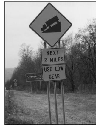
Use of too many supports, either on one sign or for a group of signs can produce a hazard. This supporting system is too rigid and may contribute to overturning, loss of control or abrupt stopping.
