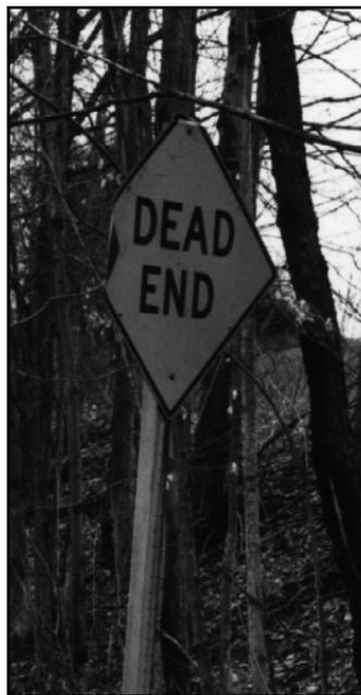
Signs may be bent like this DEAD END sign. While many bent signs can be read in the daylight, some bent signs, even signs with minor bending, are difficult to see at night because they no longer reflect the light from the vehicle's headlights back to the driver's eyes. Minor bending like this may be repaired by removing the sign from the post and straightening the sign face.
