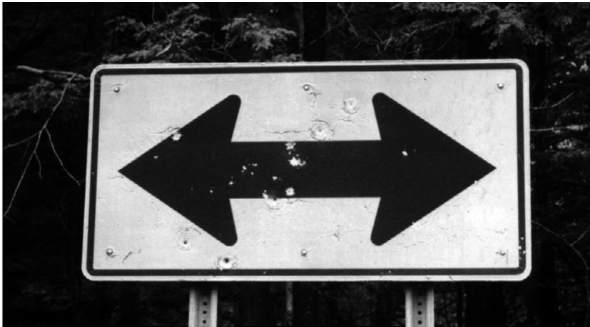
Field patching can be done by preparing a repair kit that includes the appropriate colors and types of new sheeting materials (including pressuresensitive adhesive sheeting), cleaners and sealants.
