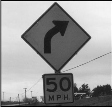
The sign face is cracking. Retroreflective surfaces that have splits, breaks, peels, or separations should be replaced as soon as practical with a new sign.
