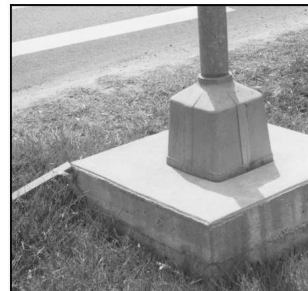
While the system used is a break-away base the pedestal it is mounted on was either not back filled around or the soil has eroded around it. This support system is now a hazard as it constitutes a rigid concrete block more than four inches above the surrounding ground. This can snag the under-carriage of a vehicle causing it to stop abruptly or go out of control.
