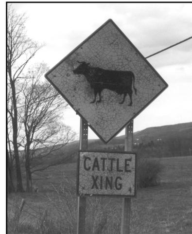
This sign is old and the surface is seriously cracked – it has lost its retroreflective characteristic and appears as a distorted image at night. If the signs are still appropriate they should be scheduled for replacement.
