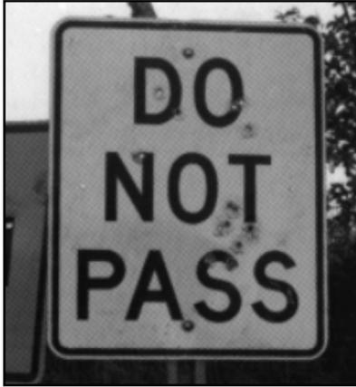
This sign has been hit by several gun shots. Even with the holes the sign can be read during the day and functions as intended, but leaving a sign up in this condition does not convey a serious message and may encourage more gun shots to this and other signs. The sign should be replaced or repaired as soon as practical.
