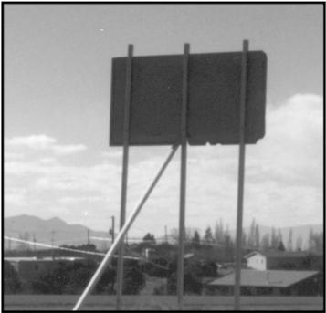
Sign supports should be repaired or replaced to original conditions. This “breakaway” support was propped up with a diagonal brace, which could affect its safe performance if it were hit again.
