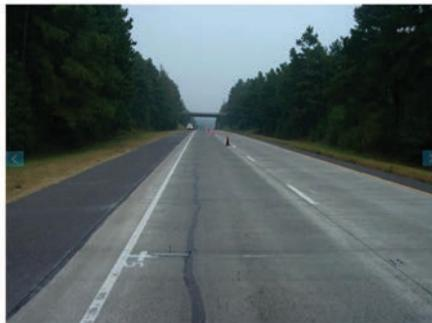
Figure 24. Longitudinal cracking near the shoulder in Arkansas-0217 section (December 4, 2012).
