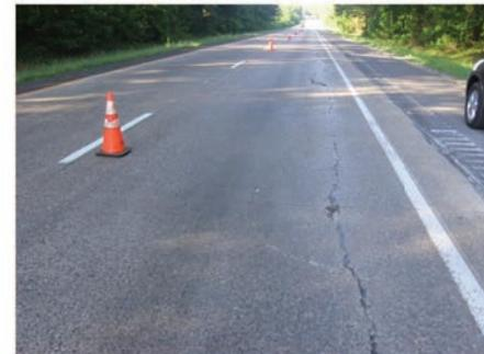
Figure 25. Longitudinal cracking near the shoulder in Colorado-0217 section (September 20, 2011).
