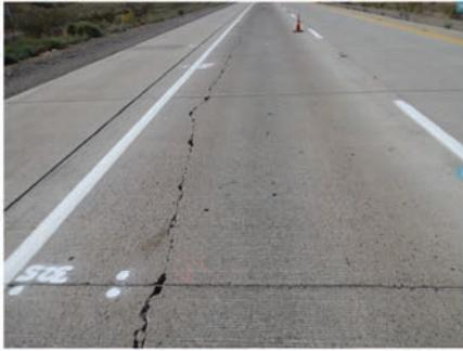
Figure 22. Longitudinal cracking near the shoulder in Arizona-0262 section (February 16, 2011).
