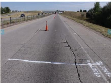
Figure 26. Longitudinal cracking near the shoulder in Colorado-0218 section (September 20, 2011).
