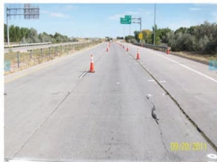
Figure 27. Longitudinal cracking near the shoulder in North Dakota-0217 section (August 21, 2012).
