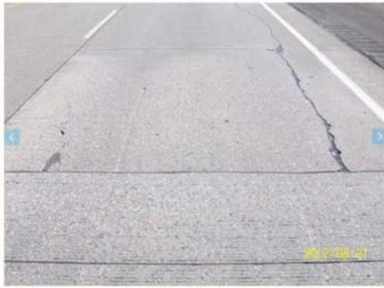
Figure 28. Longitudinal cracking near the shoulder in Iowa-0217 section (March 30, 2011).
