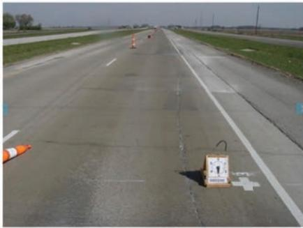
Figure 30. Longitudinal cracking near the shoulder in Washington-0206 section (May 23, 2013).
