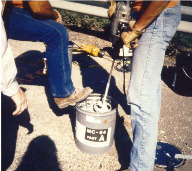
Figure 21. Using a jiffy mixer.
