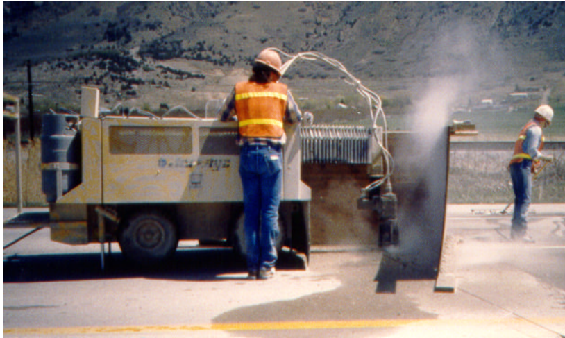
Figure 16. Protective shield around waterblasting operation.
