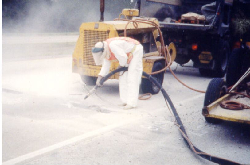
Figure 17. Sandblasting.
