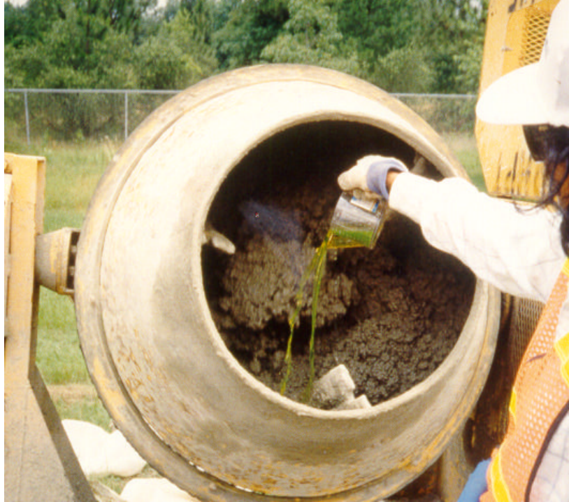
Figure 20. Adding carefully measured components to a drum mixer.
