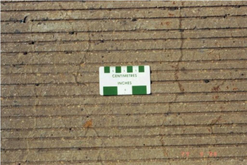
Figure 34. Cracking in 12-Year-Old Bridge Deck.
