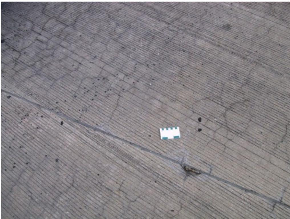
Figure 35. Cracking of 11-Year-Old Untreated Section of Rt. 1 in Delaware.
