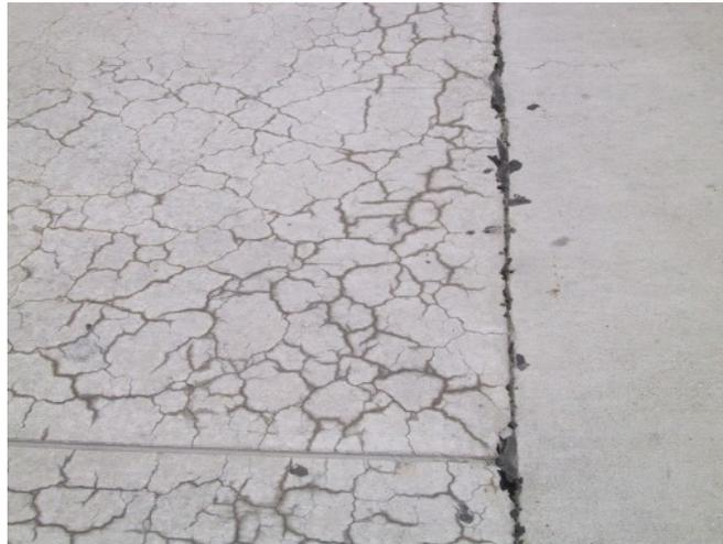
Figure 9. Extrusion of Joint-Sealing Material Triggered by Excessive Expansion Due to ASR.
