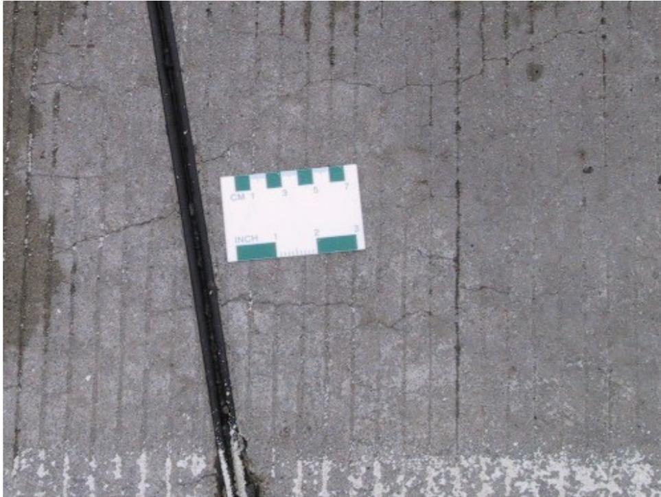
Figure 22. Lackawanna Valley Industrial Highway Experimental Pavement—15 percent Class F Fly Ash (Mix #9)—May 2001.
