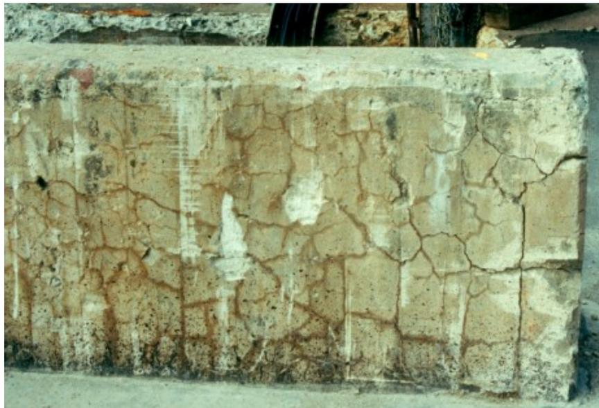
Figure 6. ASR-Induced Damage in Unrestrained Concrete Element. Uniform Expansion in All Directions Results in Classic Map-Cracking.
