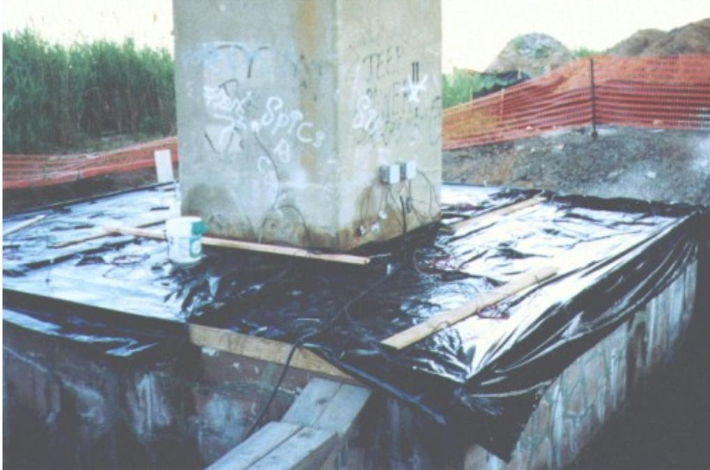
Figure 39. Application of an Electrochemical Lithium Migration Technique for a Pier Footing on the New Jersey Turnpike.
