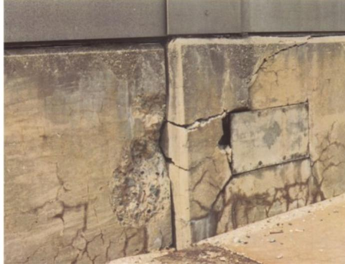
Figure 8. Misalignment of Adjacent Sections of a Parapet Wall on a Highway Bridge Due to ASR-Induced Expansion (Strategic Highway Research Program (SHRP)-315, 1991).
