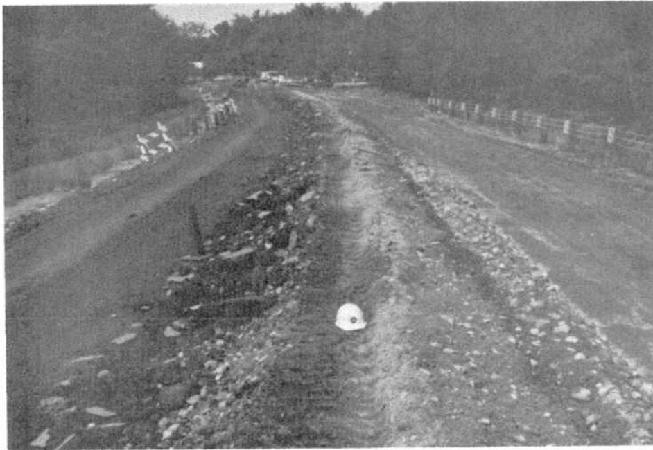
FIGURE T-7: Center Windrow with Partial Placement of Crushed Gravel (Looking South)
