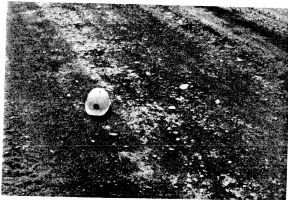
FIGURE T-14: Completed Reclaimed Stabilized Base (Note Consolidation of Material)
