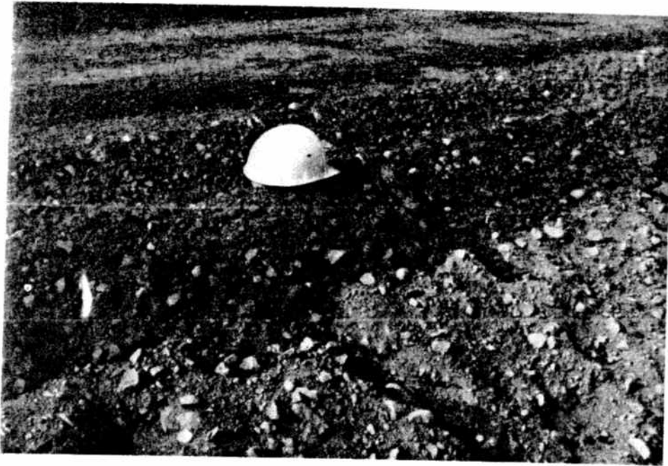
FIGURE T-13: Completed Reclaimed Stabilized Base
