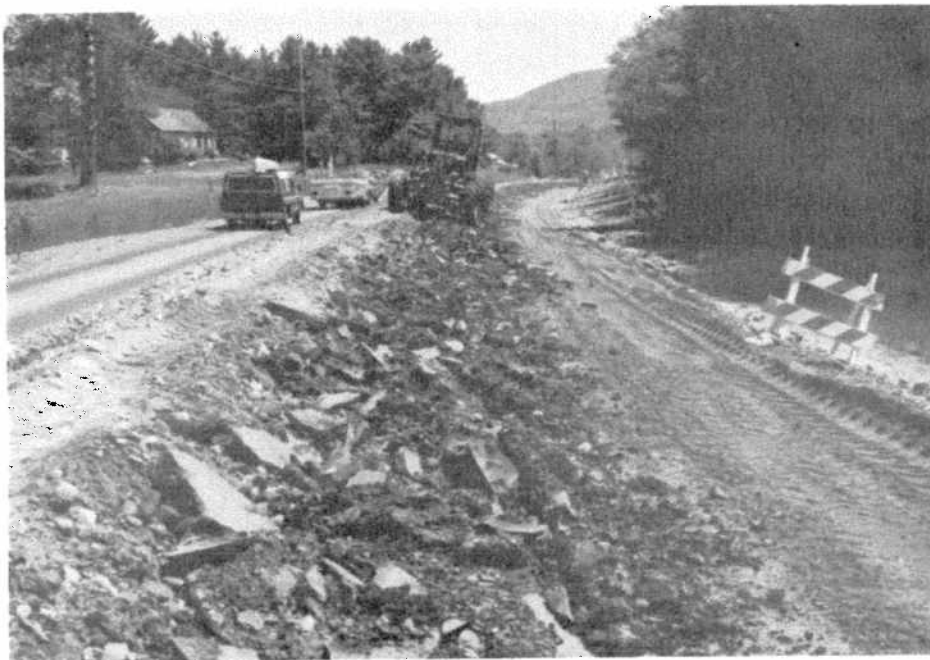
FIGURE T-7: Center Windrow with Partial Placement of Crushed Gravel (Looking South)
