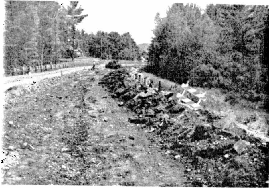
FIGURE T-9: Material Being Crushed and Bladed (Looking North)
