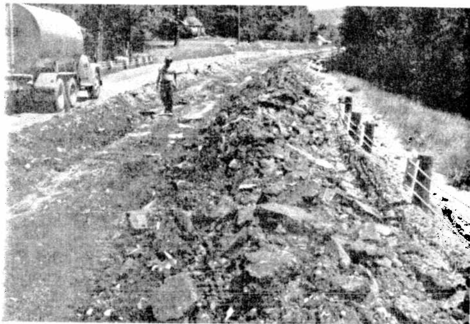
FIGURE T-9: Material Being Crushed and Bladed (Looking North)
