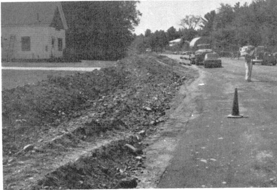
FIGURE T-11: Windrow Completed (Looking South)
