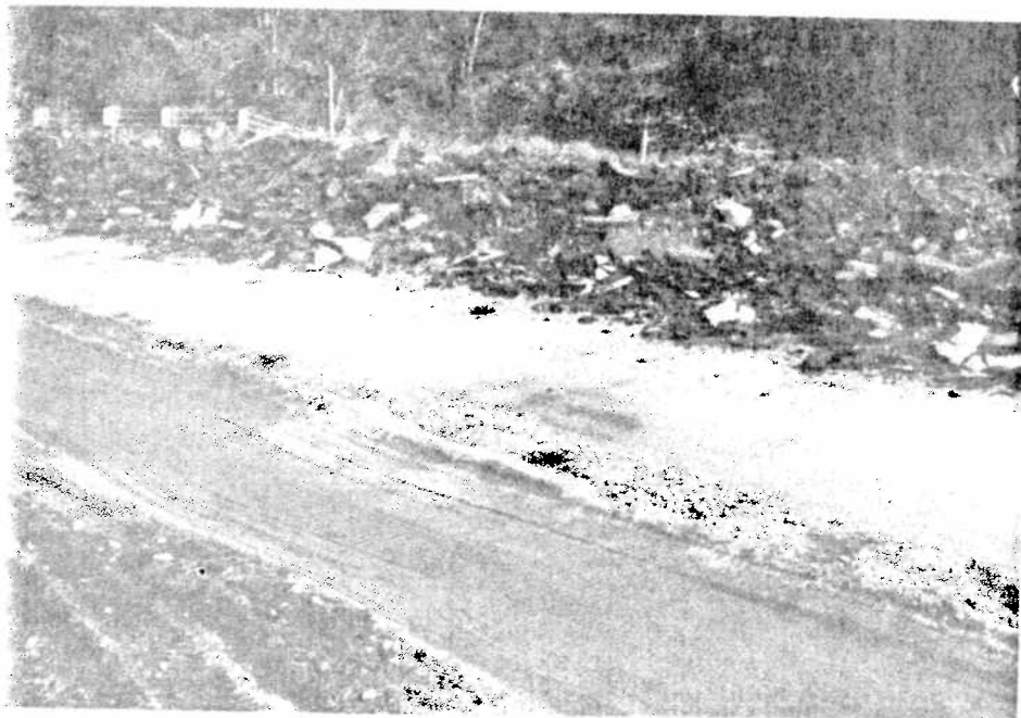
FIGURE T-6: One-Way Detour and Center Windrow of Crushed Pavement
