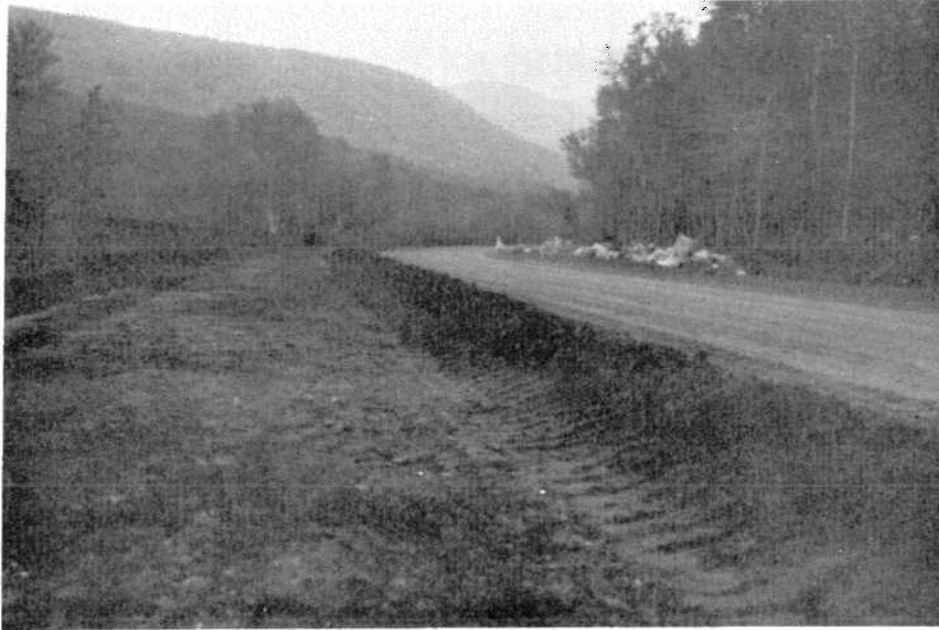
FIGURE J-13: Small Windrow Graded to Center Prior to Hammermilling Operation (Looking South)
