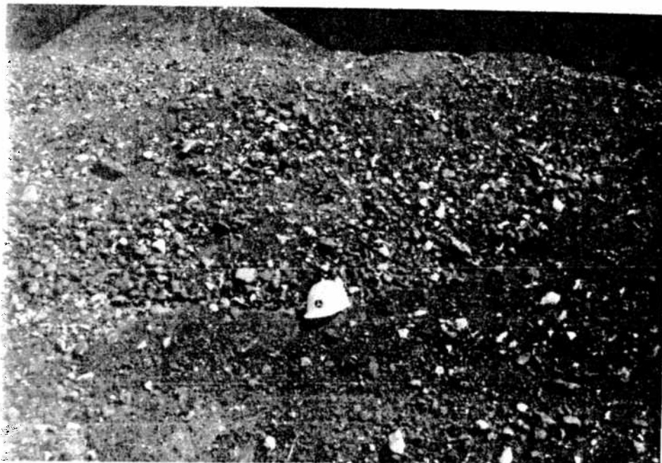
FIGURE J-6: Reclaimed Material Stockpile (After In-Place Crushing, Prior to Hammermill Operation)
