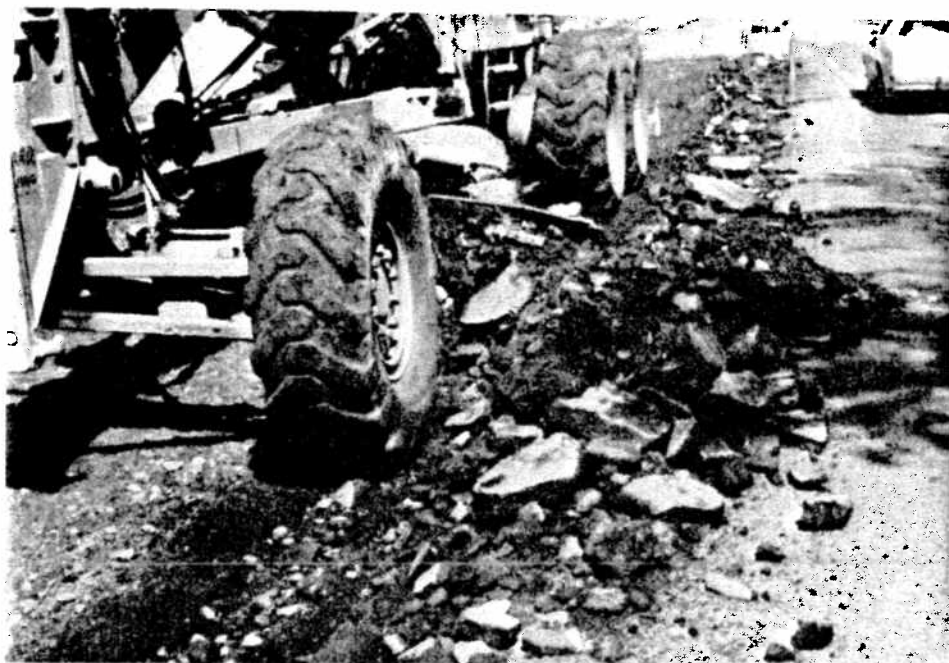
FIGURE J-2: Existing Pavement Broken Up After Use of Ripper Tooth
