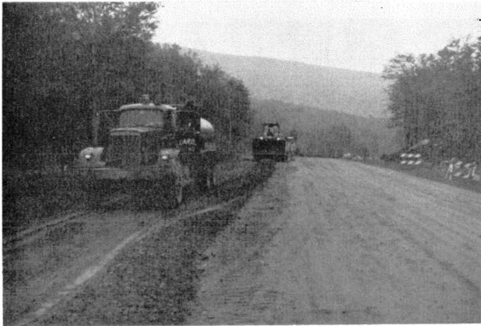
FIGURE J-14: Water Applied to Windrow (Looking South)
