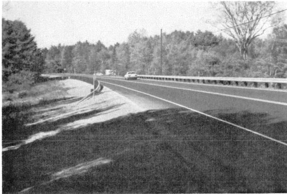
FIGURE T-15: Completed Project (Same View as T-7 and T-12)
