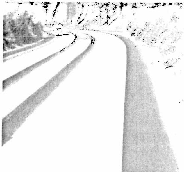
Completed Recycled AC Shoulders Figure 24
