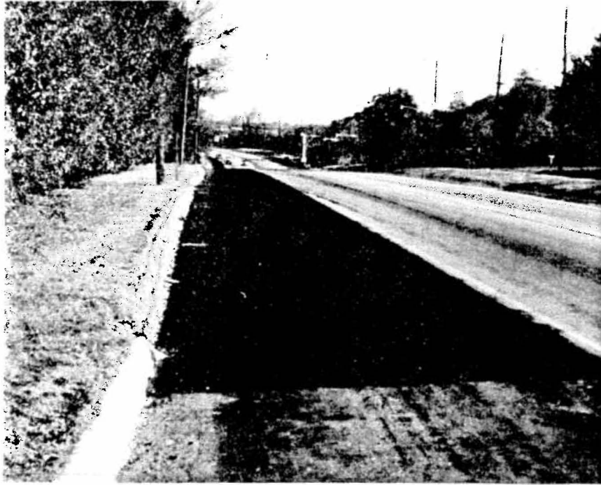
FIGURE 17 Finished Shoulder Pavement
