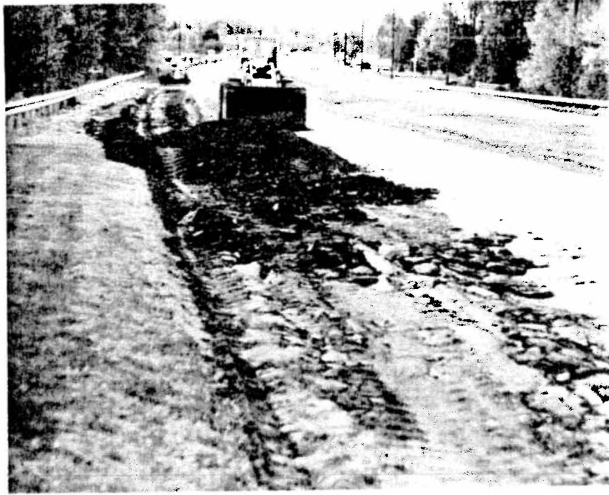
FIGURE 11 Shoulder Excavation
