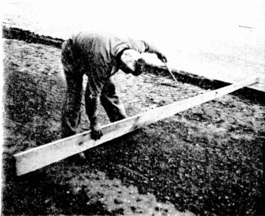
FIGURE 14 Checking Grade
