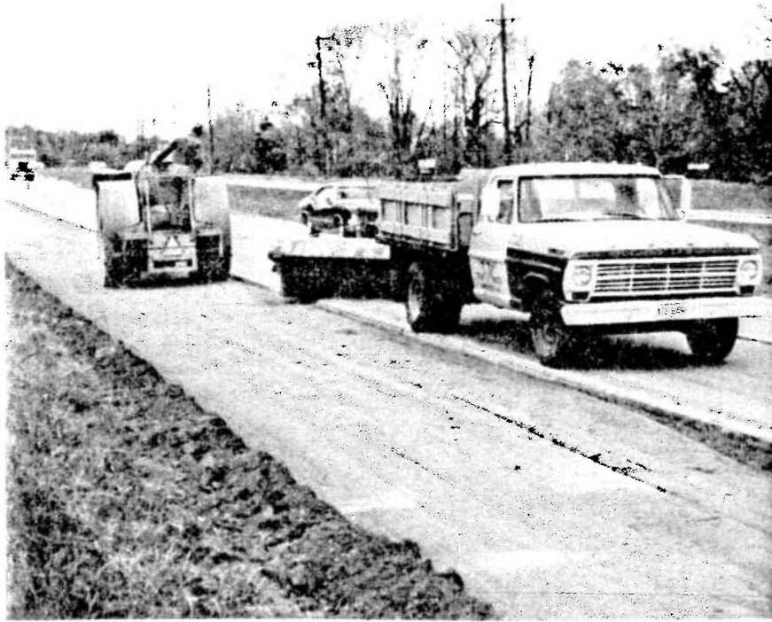
FIGURE 13 Compacting
