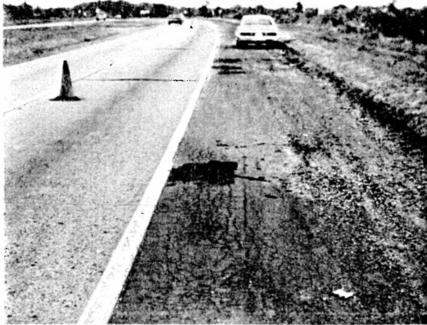
FIGURE 10 Shoulder before Recycling
