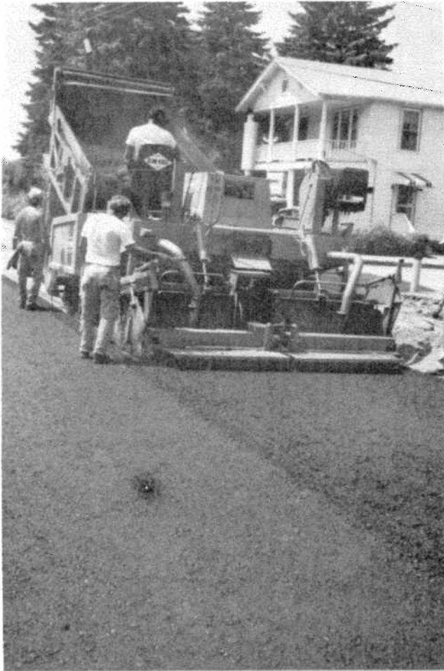
FIGURE M-10: Placement of Recycled Material on Second Street
