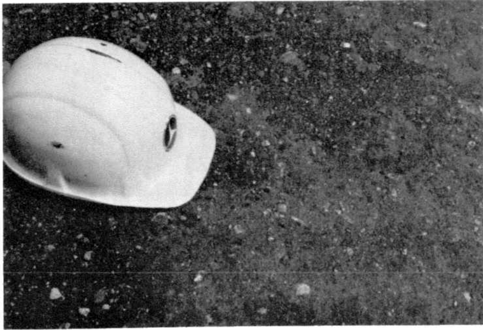
FIGURE C-4: Surface at Maintenance Yard Prior to Application of Penetrating Oil
