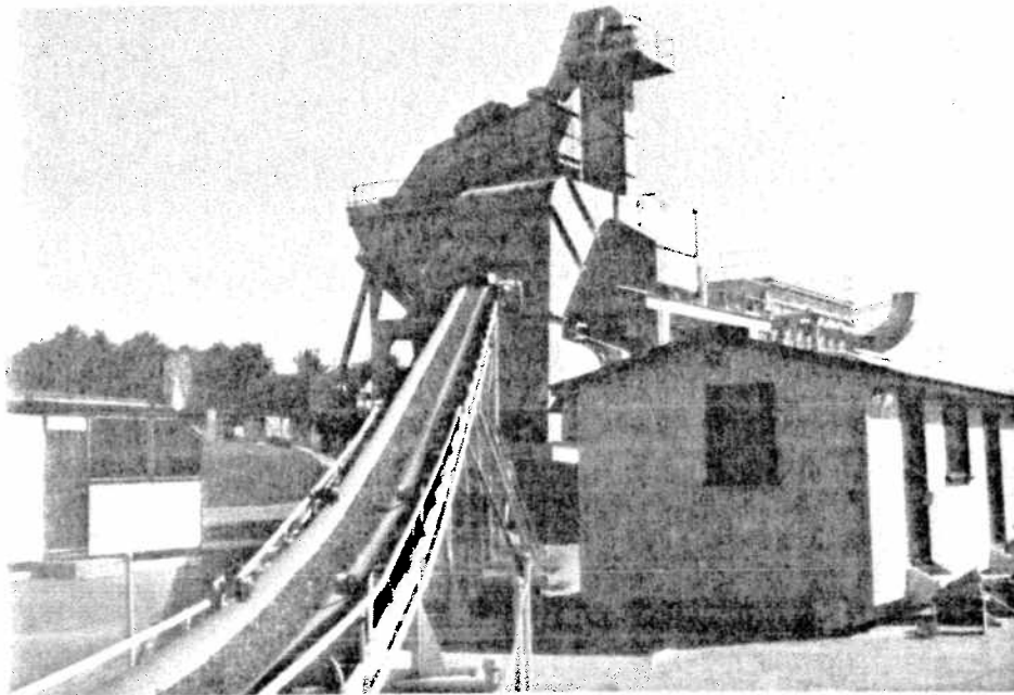
FIGURE C-10: Conveyor from Virgin Aggregate Bins to Dryer. Left Background: Control House
