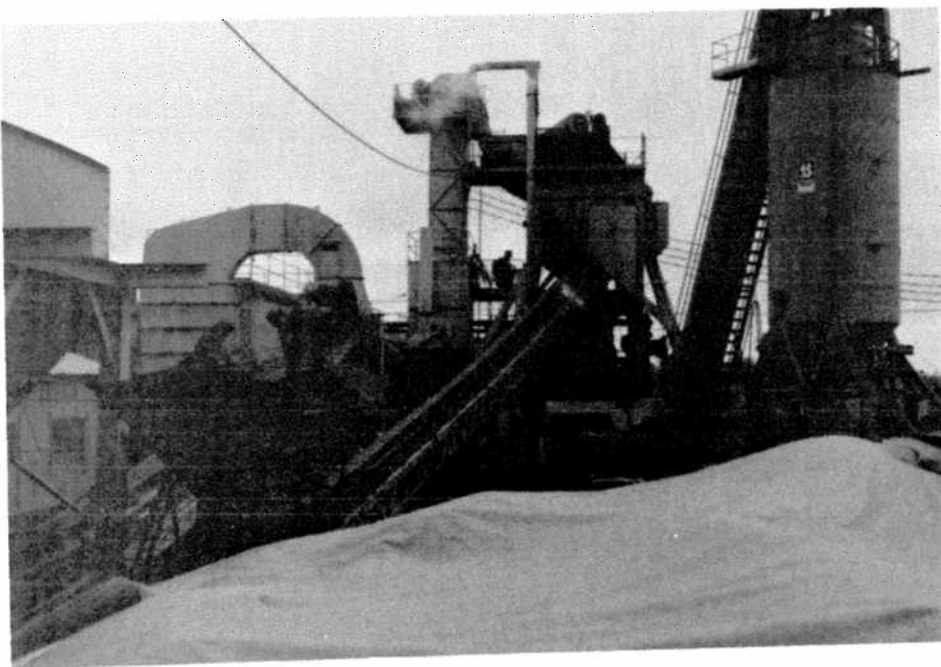
FIGURE M-9: Asphalt Batch Plant. In foreground extreme left, virgin aggregate bins with conveyor. In foreground recycle bin with conveyor; in background, dryer. Off center to the right is the central batch plant with asphalt storage tank.
