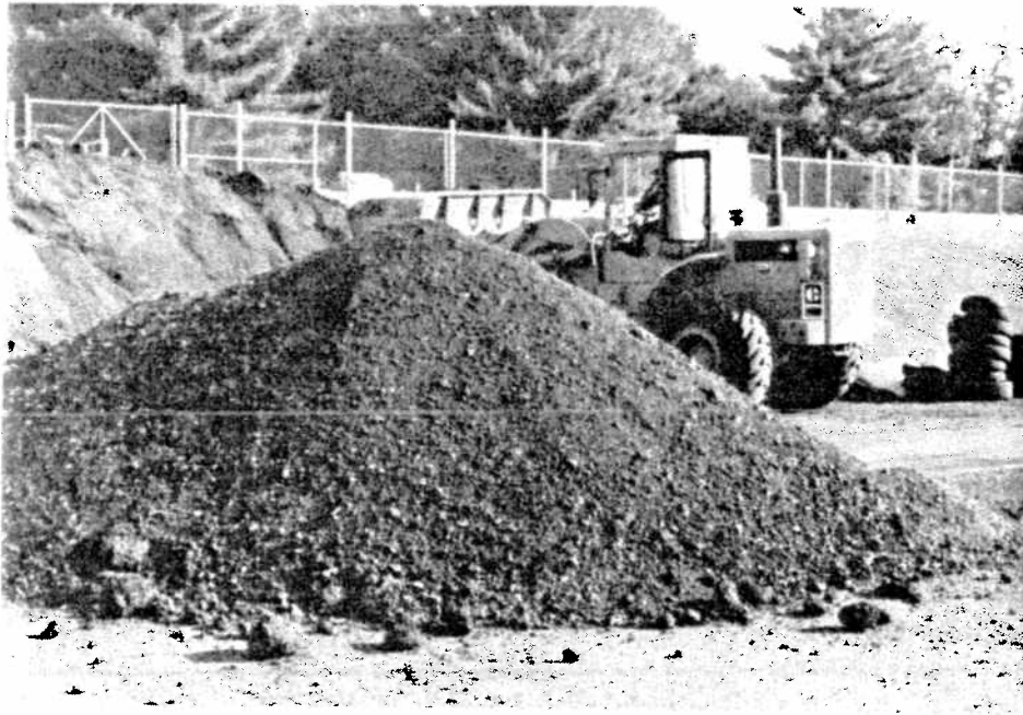
FIGURE C-5: Blending of Milled Material Stockpile at Plant Site
