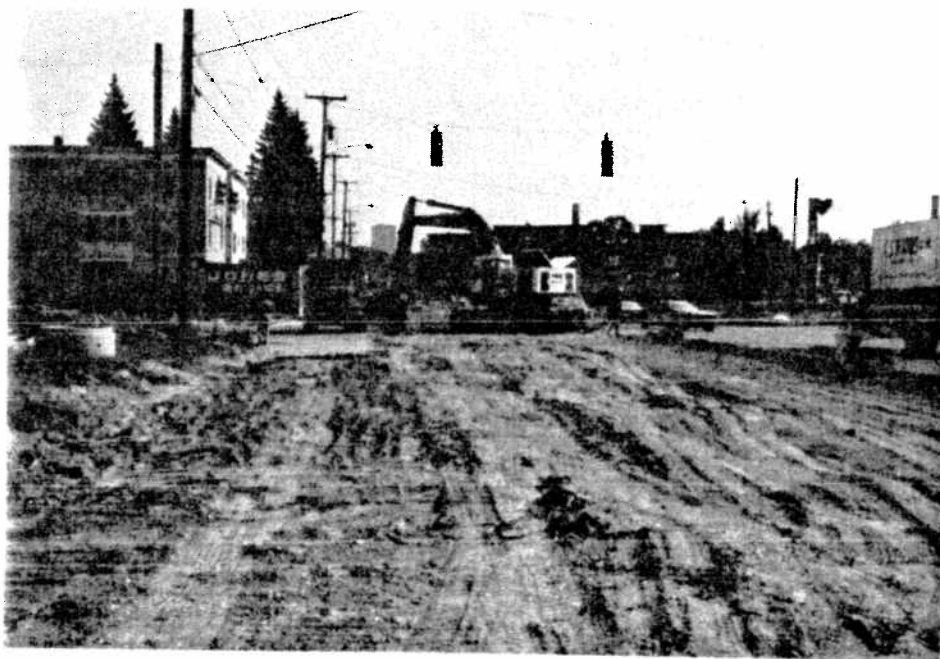
FIGURE M-3: Removal of Existing Pavement for Recycling
