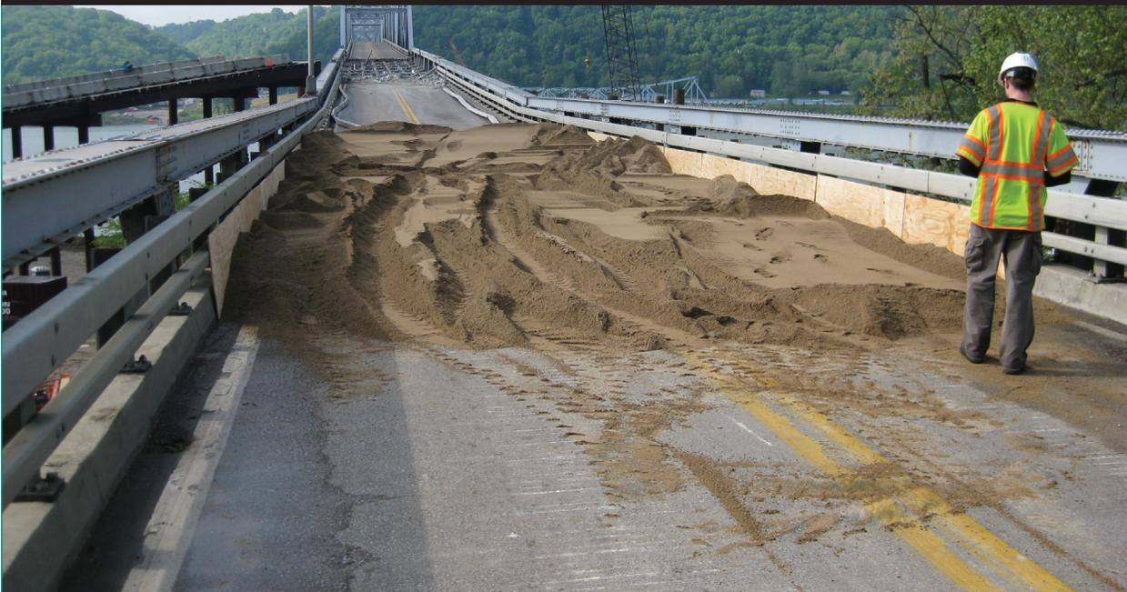
Figure 6. Shape charges applied to one web plate of chord member.
