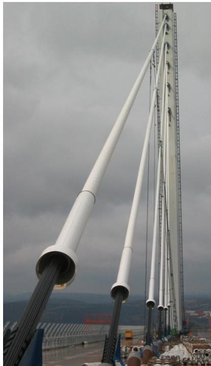
**Figure 1. Photo. Modern stay cables with HDPE tube cover on the Millau Viaduct.**
