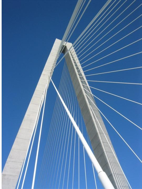
**Figure 2. Photo. Modern stay cables with HDPE tube cover on the Clark Bridge.**
