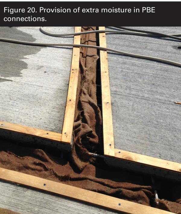
Figure 20. Provision of extra moisture in PBE connections.
