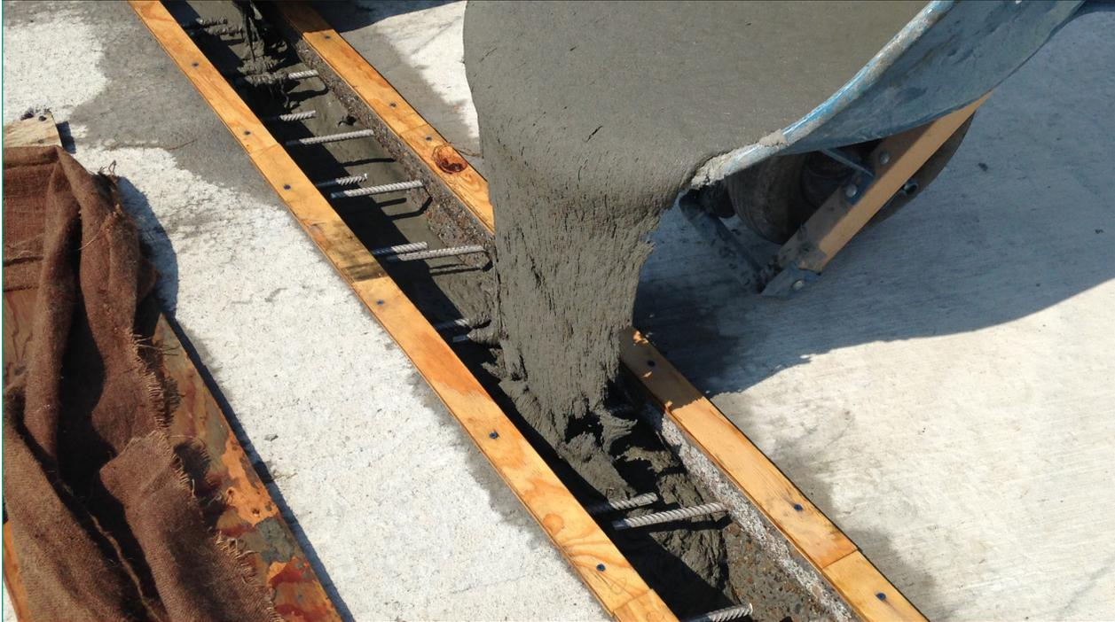
grouts that employ alternative binder systems (e.g., micro-silica) with or without the use of fiber reinforcements.
