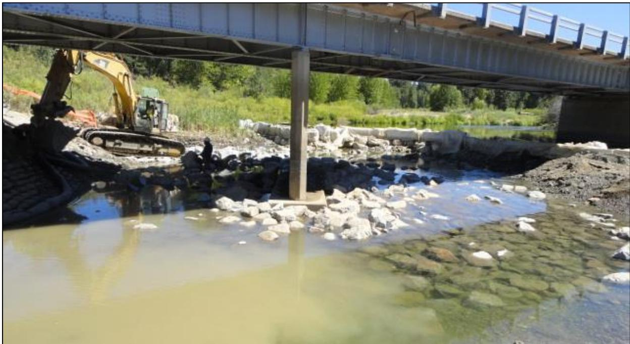
**Figure 27. Photo. Riprap installation near pier 3 (August 2012).**
