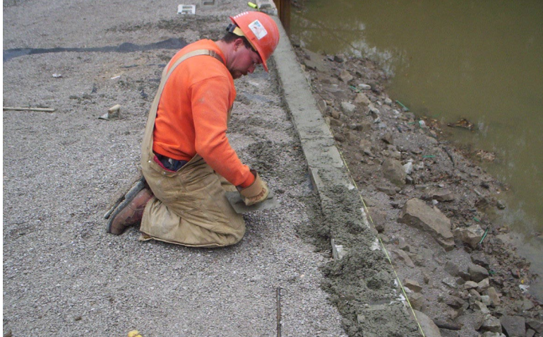
Figure 74. Photo. Connecting the top courses of blocks.
