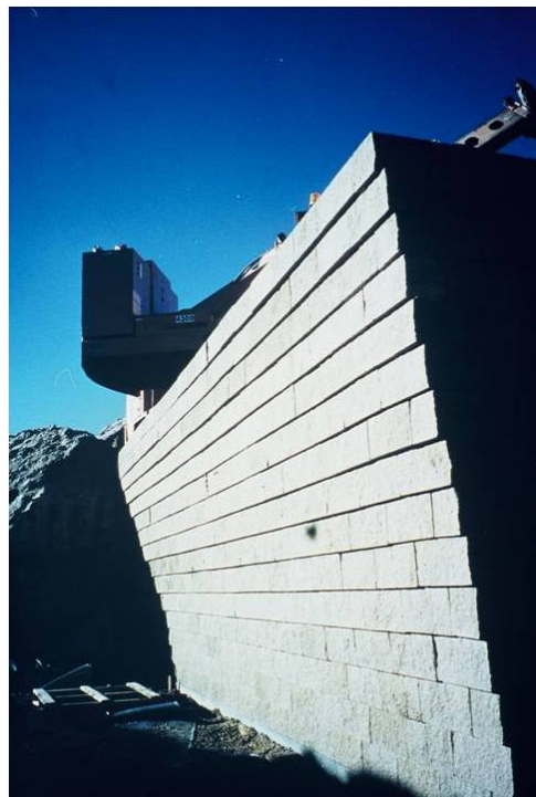
Figure 64. Photo. Negative batter wall face.
