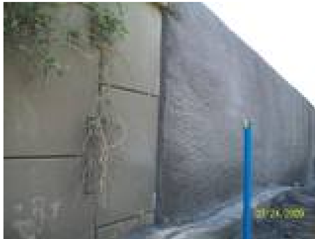
Figure 106. Photo. Use of GRS wall to repair damaged MSE wall.
