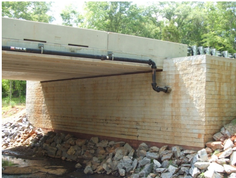
Figure 100. Photo. Utilities through a GRS abutment.
