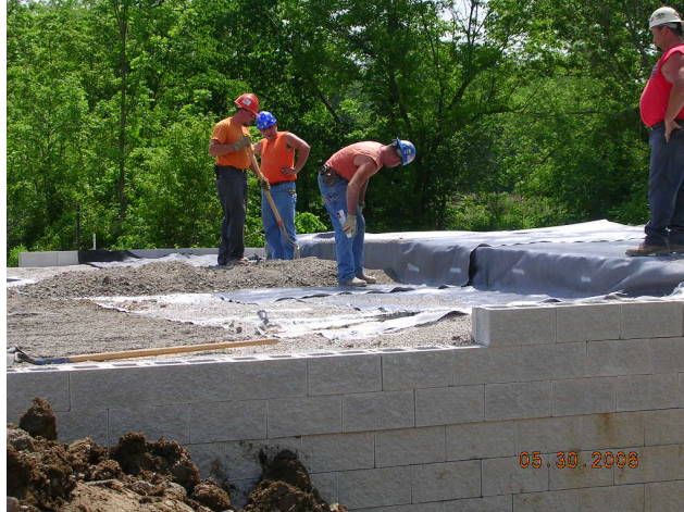
Figure 93. Photo. First 6-inch-thick fill lift.
