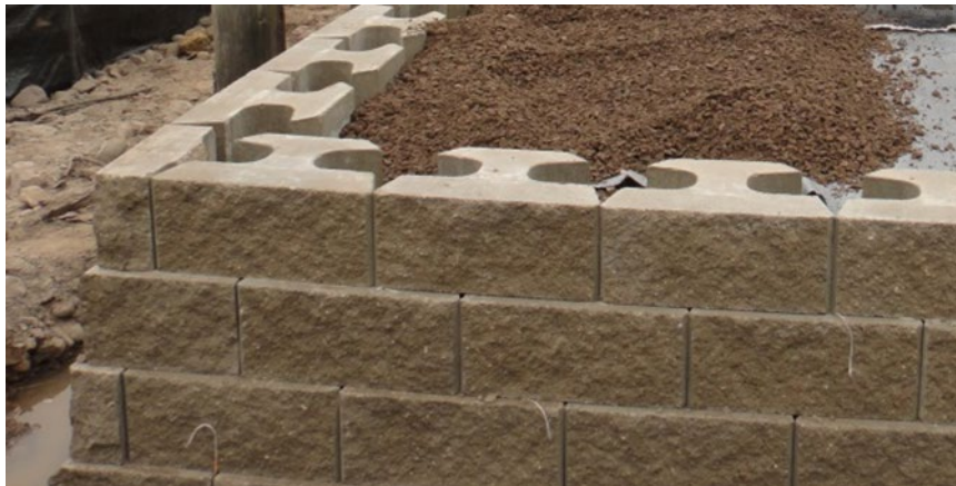
Figure 10. Photo. GRS abutment constructed with an SRW block facing.
