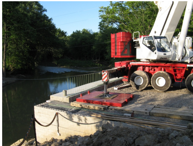
Figure 89. Photo. Outrigger pads near the wall face.
