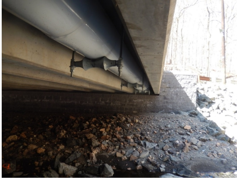
Figure 100. Photo. Utilities through a GRS abutment.
