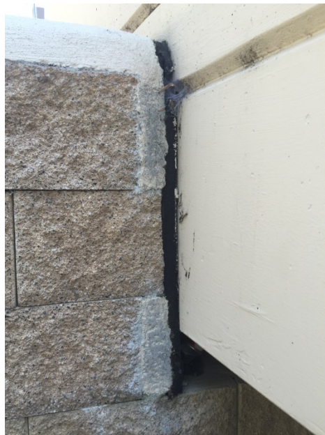
Figure 104. Photo. Repair of damaged block with colored mortar.
