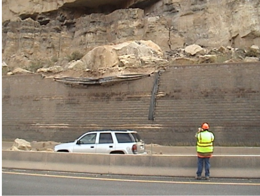
Figure 108. Photo. GRS wall damaged by a large sandstone boulder.
