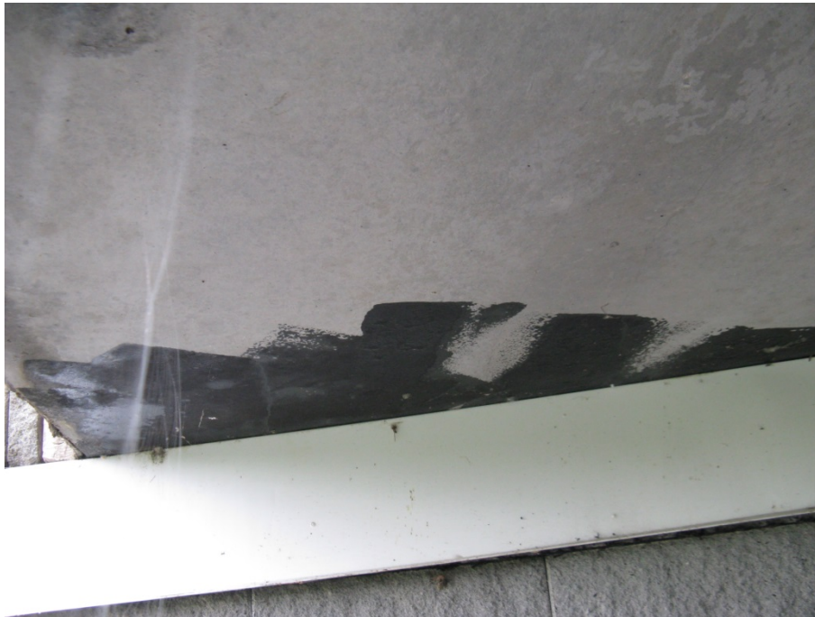
Figure 13. Photo. Bitumen coating under voided slabbeam.
