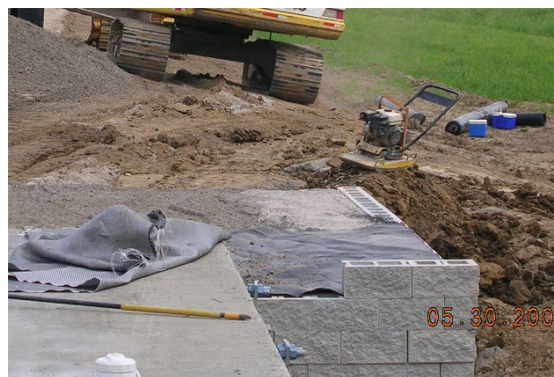
Figure 91. Photo. Second view of parapet and wing wall construction.
