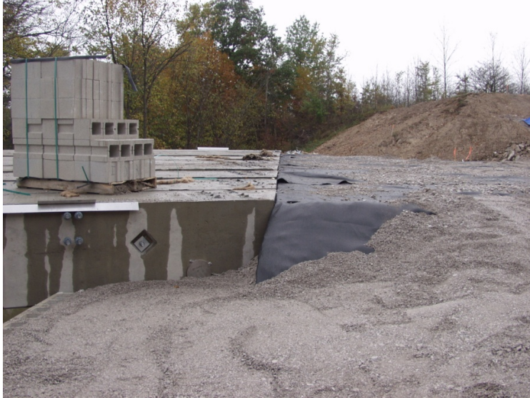
Figure 97. Photo. Completed approach fill.
