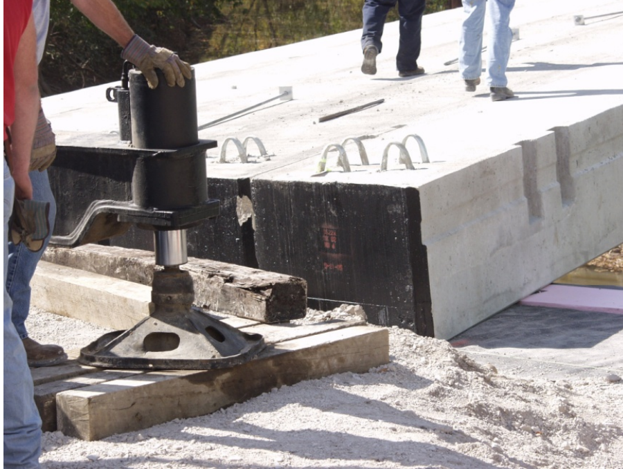
Figure 12. Photo. Bitumen coating on concrete beam ends.
