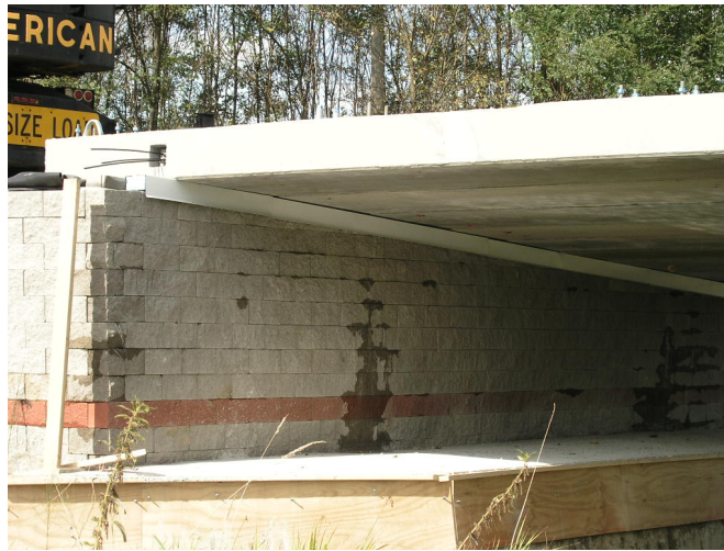
Figure 85. Photo. Aluminum flashing (drip edge) between the beams and the top of the CMU facing.
