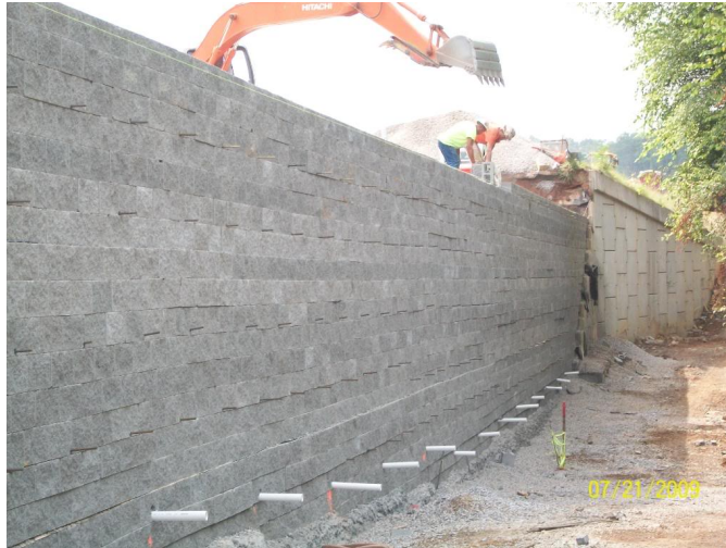
Figure 106. Photo. Use of GRS wall to repair damaged MSE wall.
