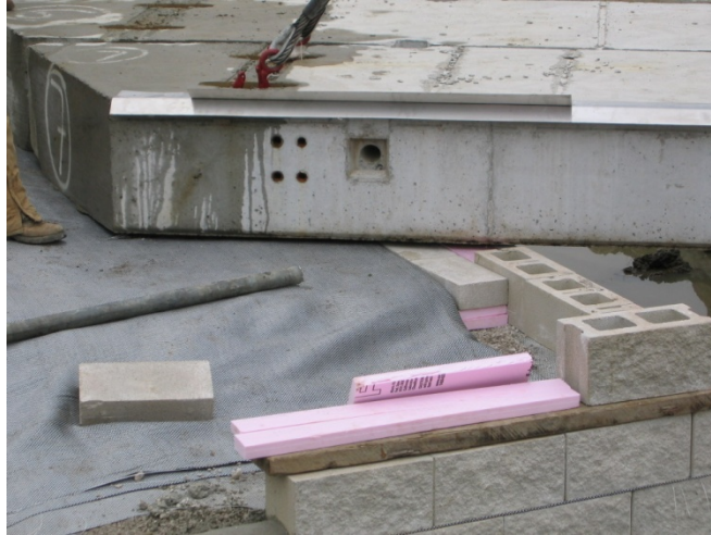
Figure 83. Photo. Top 4-inch wrap butted against a 4-inch solid block.
