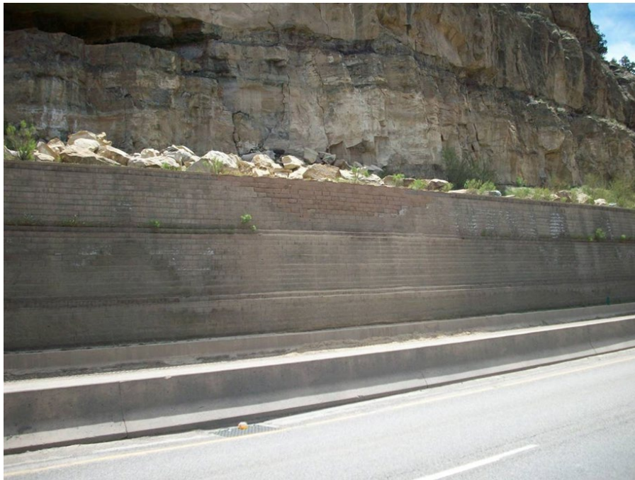
Figure 109. Photo. Repair of a GRS wall after damage caused by rock fall.
