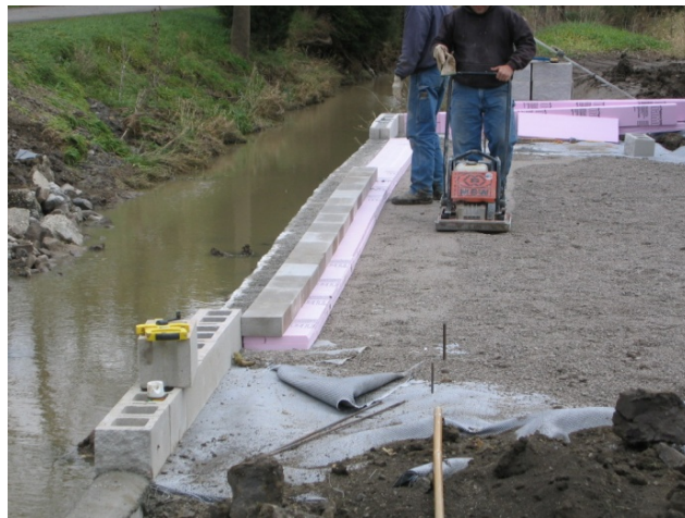
Figure 80. Photo. Foam board and 4-inch-thick block assembly to form a beam seat.
