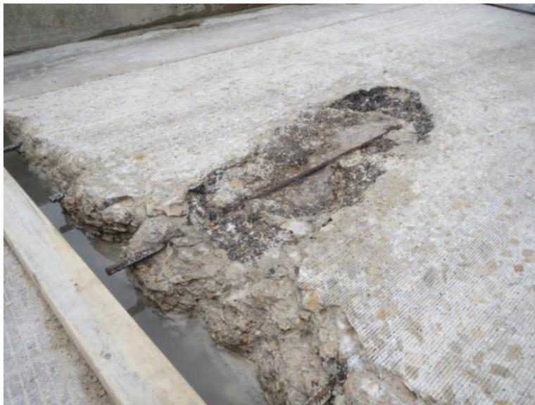
**Figure 17. Photo. Distressed region observed on the westbound lane near west abutment prior to installing the UHPC overlay.**
