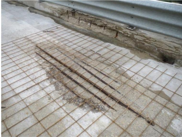
**Figure 16. Photo. Distressed region observed on the westbound lane over the pier 1 prior to installing the UHPC overlay.**
