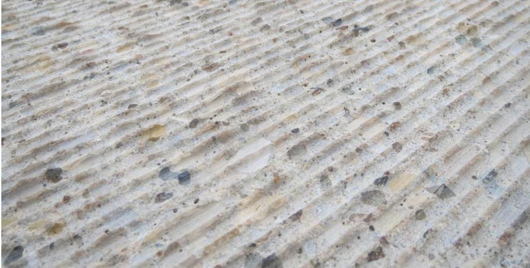
**Figure 18. Photo. Deck surface after scarification.**
