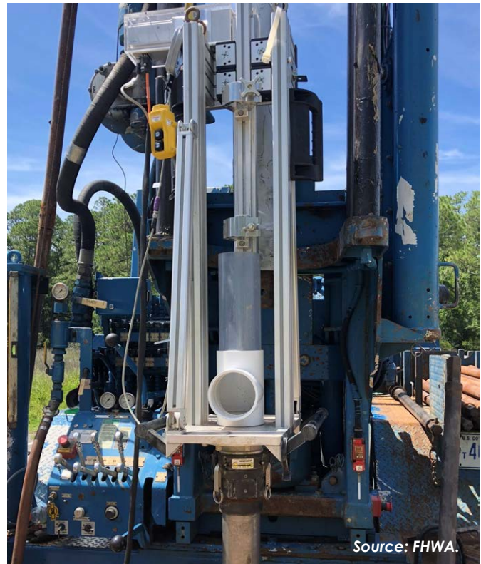
The advanced linear drive mounted on steel casings in front of the drill rig.
