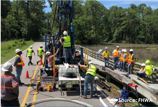
Hydraulics team assembling ISTD equipment at Gulf Islands National Seashore.
