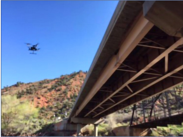
Figure 13. Photo. Glenwood Springs Bridge structural members being imaged by a UAS.
