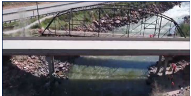
Figure 12. Photo. UAS image of the Glenwood Springs Bridge and surrounding terrain.
