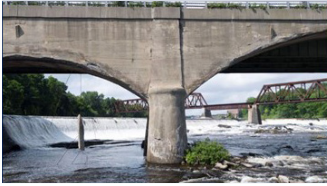
Figure 2. Photo. UAS image of Ticonic Bridge spandrel arches.
