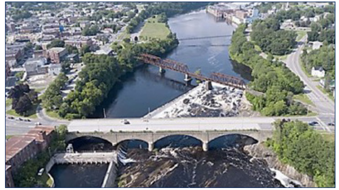
Figure 1. Photo. UAS aerial view of the Ticonic Bridge.
