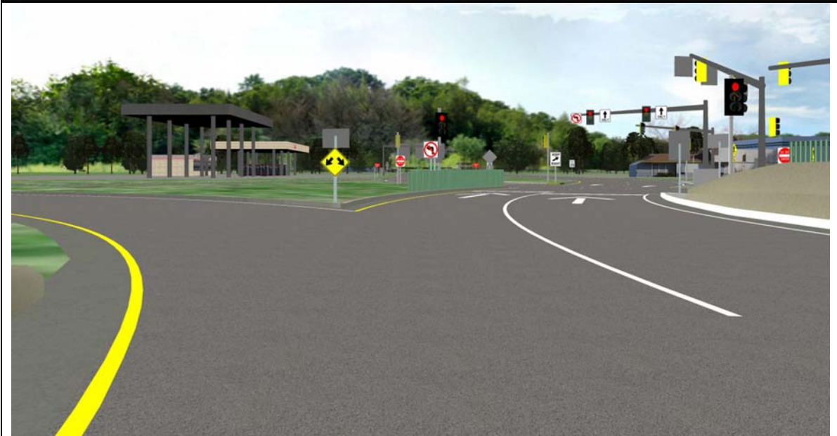
Figure 5. The approach to the free left-turn onto the northbound onramp is shown.
