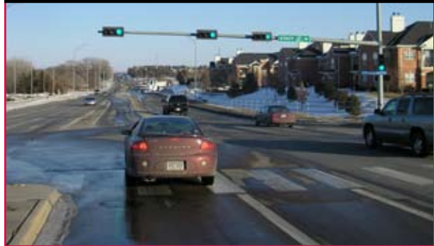
Figure 3. Example of a type 2 installation in Lincoln, NE (lateral separation with no offset).
