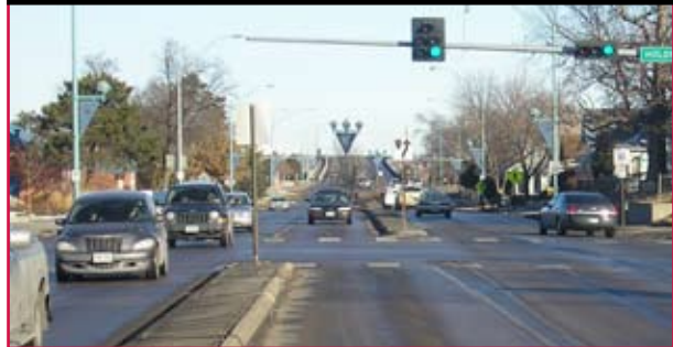
Figure 4. Example of a type 3 installation in Lincoln, NE (lateral separation with negative offset).
