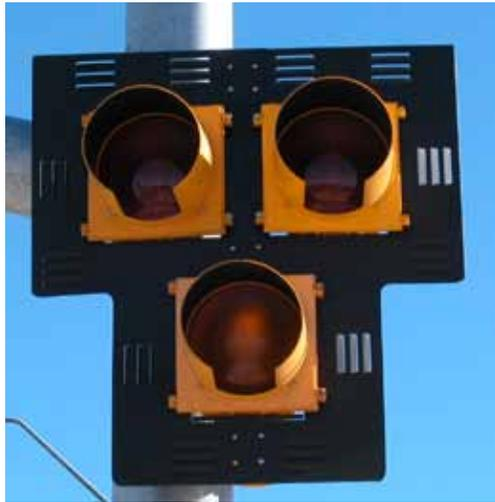
**Figure 1. Photo. Example of a HAWK head.**
