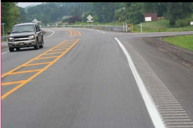
the lane width without changing the placement of the rumble strip. An alternative method for increasing the effective lane width is to use a wider edge line and place the shoulder rumble strips closer to the shoulder.
