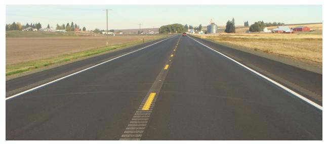
Figure 1. Photo. Combination of milled of CLRSs and SRSs.
