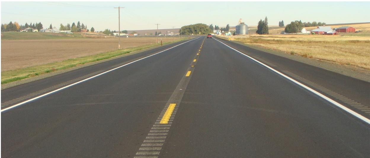
**Figure 1. Photo. Combination of milled of CLRSs and SRSs.**
