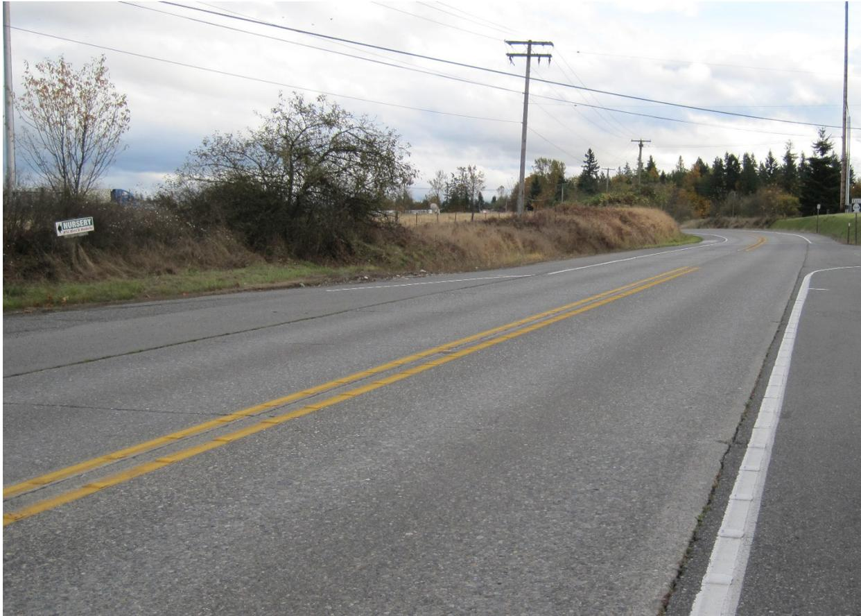
**Figure 3. Photo. Example of profiled thermoplastic pavement marking.**
