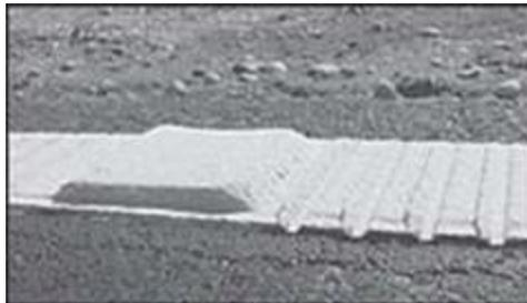
**Figure 1. Photo. Raised profiled thermoplastic marking.**<sup>(1)</sup>
