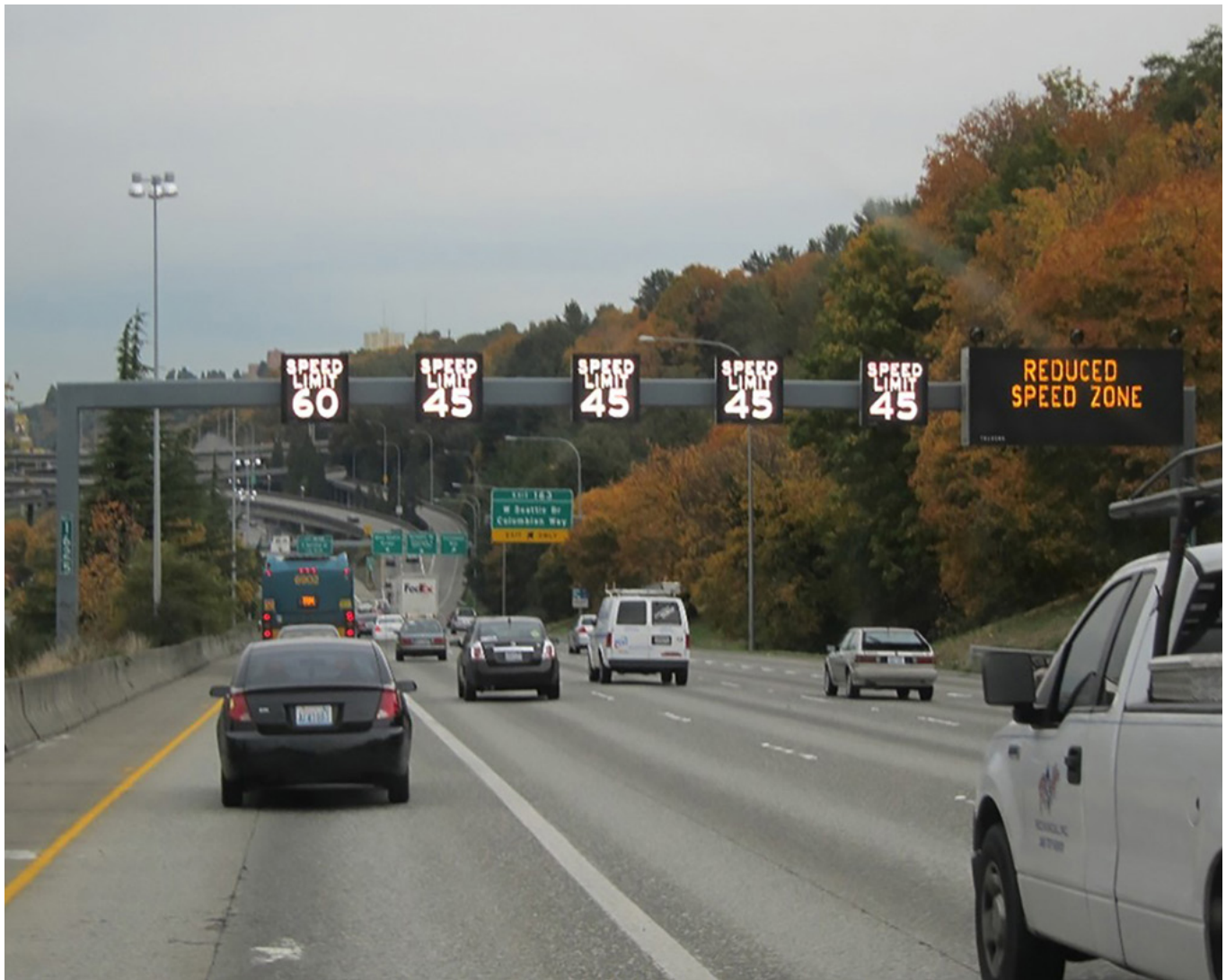
Figure 1. Photograph. VSLs on I-5 in Seattle, WA.
