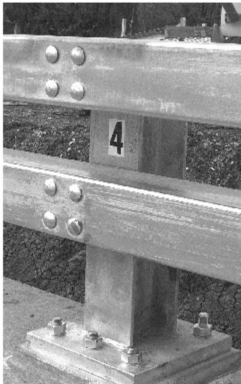
Figure 3. New York Two-Rail Curbless Bridge Railing before test 404531-2.
