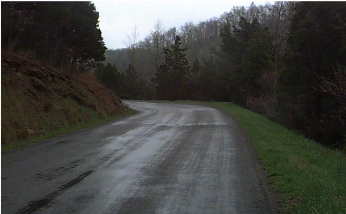
**Figure 12. Event 15: Unmarked reverse curve.**
