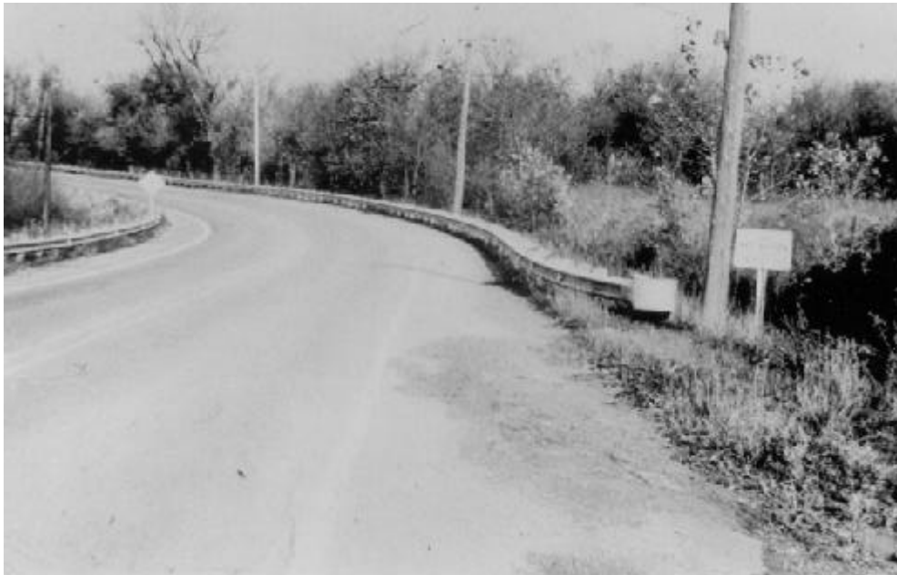
Figure 11. Typical Roadway with Roadside Hazard Rating Equal to 4.
