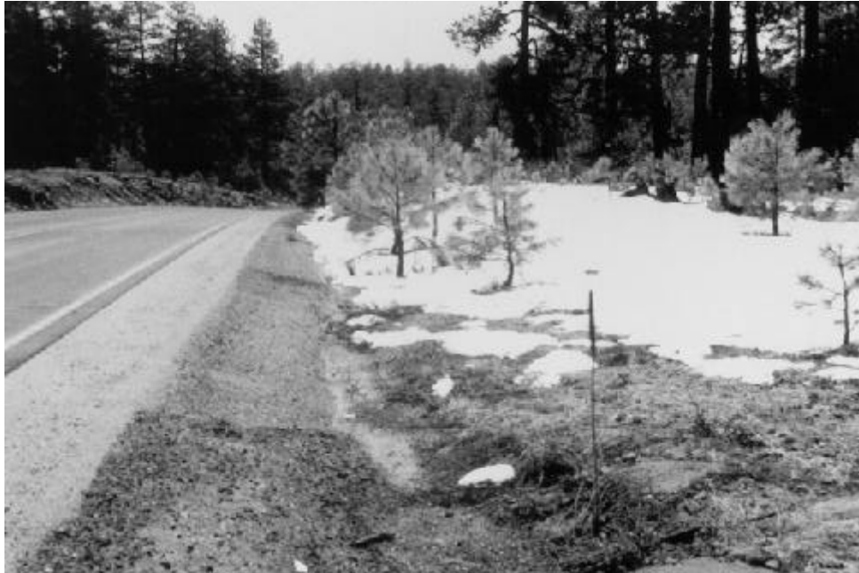
Figure 10. Typical Roadway with Roadside Hazard Rating Equal to 3.
