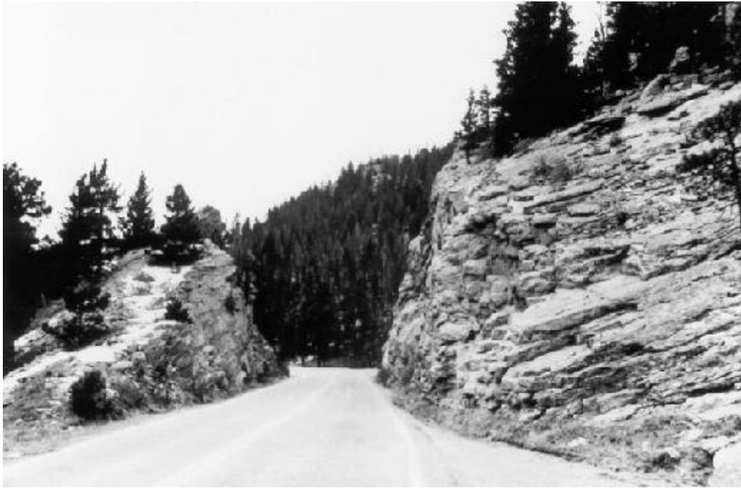
Figure 14. Typical Roadway with Roadside Hazard Rating Equal to 7.
