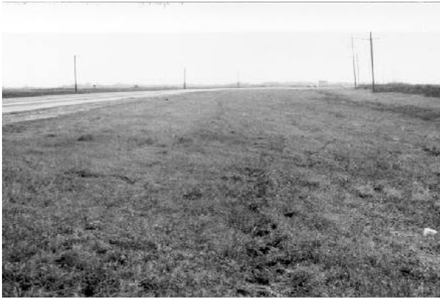
Figure 8. Typical Roadway with Roadside Hazard Rating Equal to 1.
