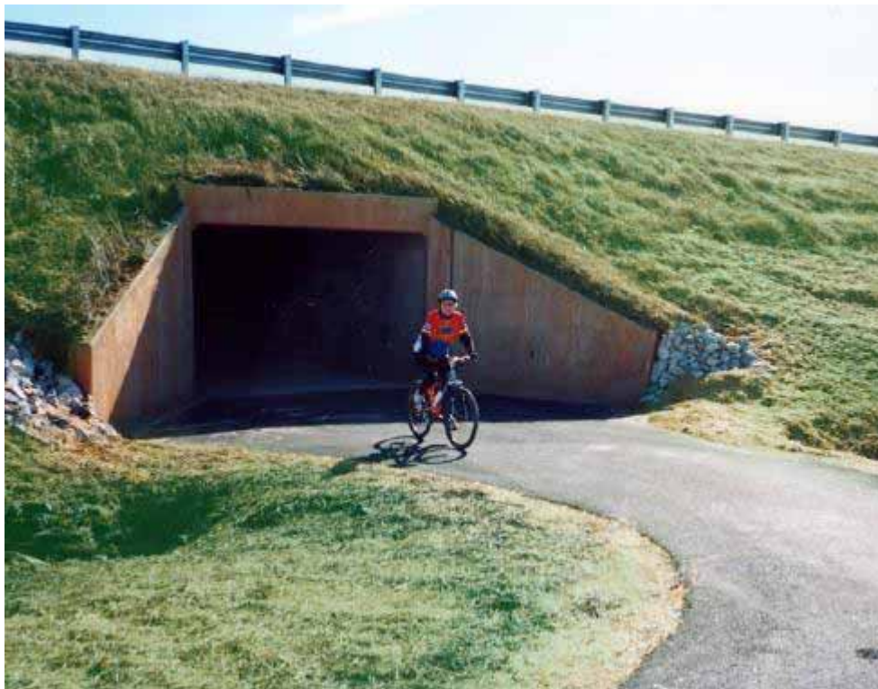
Figure 12-9. Photo. An underpass continues this shared-use bicycle path beneath a four-lane highway with high traffic volume.
