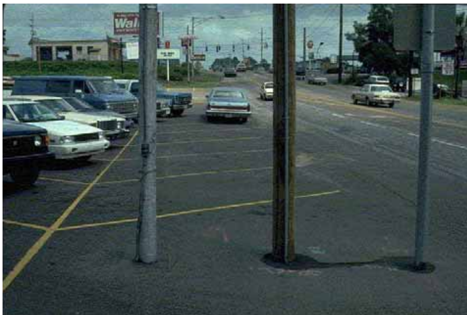
Figure 7-2. Photo. Parked cars and a lack of sidewalks along the road's edge create unsafe conditions for bicyclists and pedestrians.
